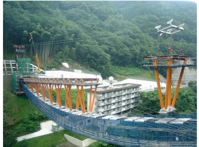
Figure 6. Installation of precast member using suspension cables.
