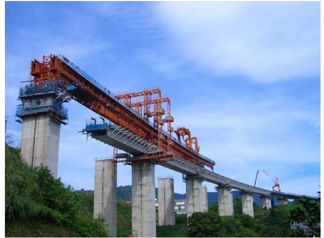
Figure 18. Precast segment cantilevering with erection girder.
