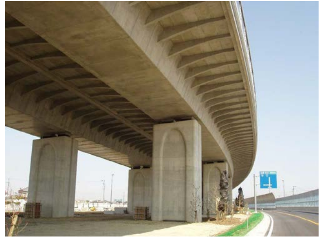
Figure 9. Furukawa Viaduct with factory fabricated segments.
