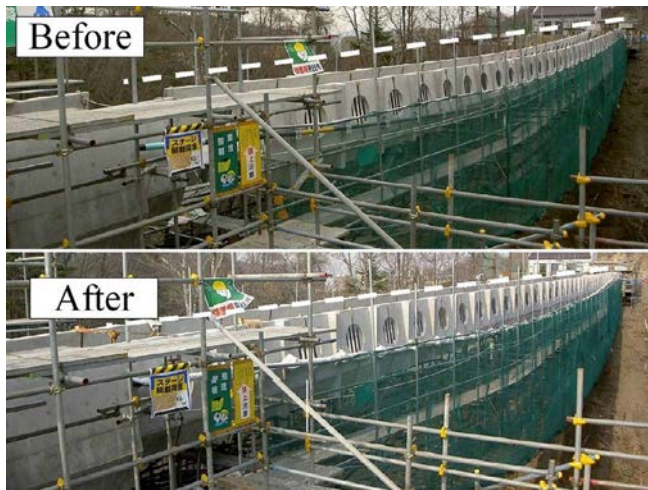
Figure 21. Adjustment of girder alignment using secondary cables.
