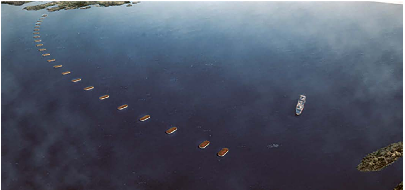
Figure 7. Study for an SFTB with pontoons for the Bjørnafjord crossing in Norway, Statens vegvesen.
