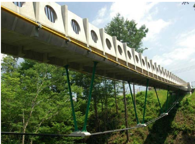
Figure 19. Seishun Bridge with double suspension cables.
