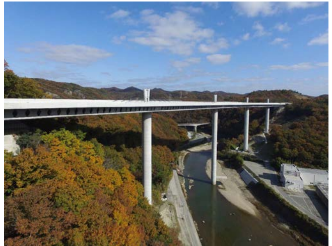
Figure 22. Mukogawa Bridge with lightweight structure.
