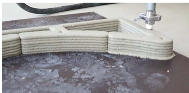
Figure 4. Anchorage details of 3D concrete printed shell element including tensile FRP reinforcement during the 3D concrete printing process (Lab. of Construction Materials and Technologies, BME, Budapest) (Photo GL Balázs).
