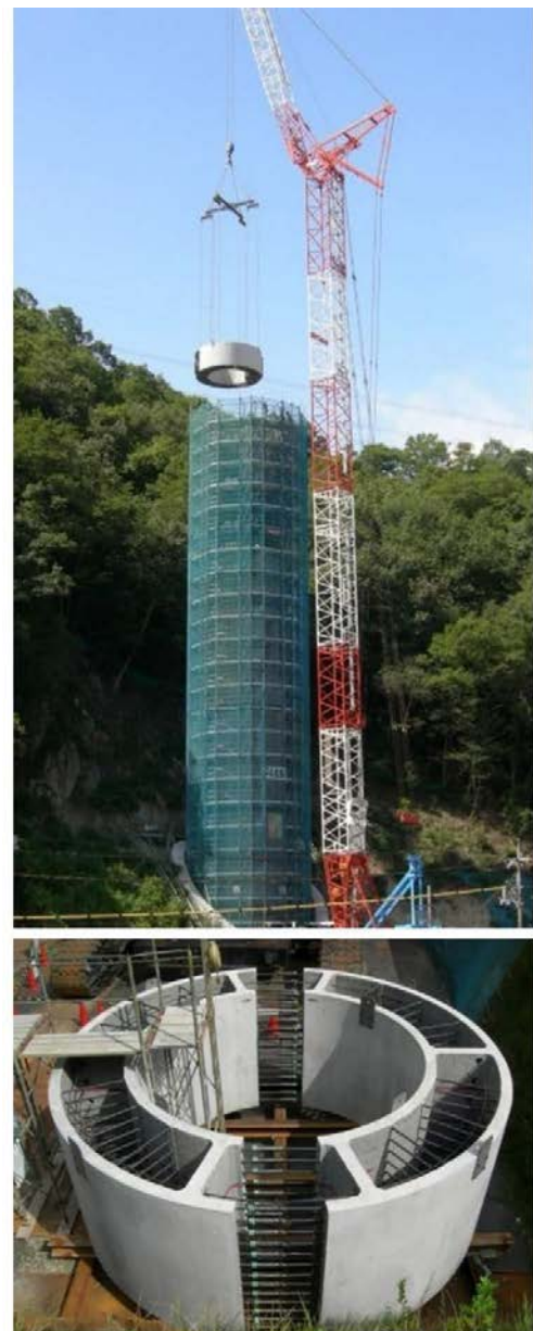
Figure 23. Half precast erection of 80m high pier.
