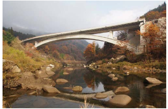
Figure 13. Kakehashi Ichigou Bridge with concrete arch.
