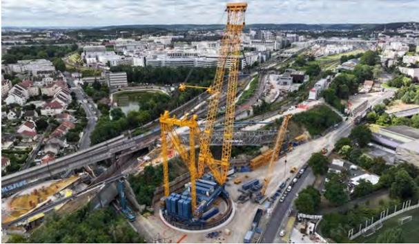
Figure 1. Lifting of old Gallardon Bridge – Old Chartres Bridge moving to demolition area.
