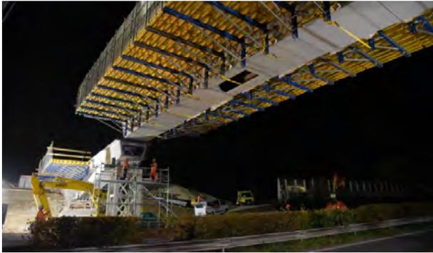
Figure 1. Main span lifting and installation.
