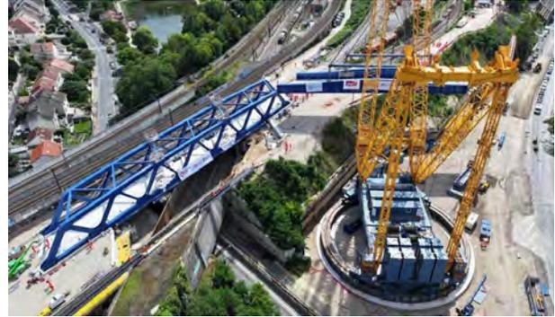
Figure 2. Lifting of new Chartres bridge.
