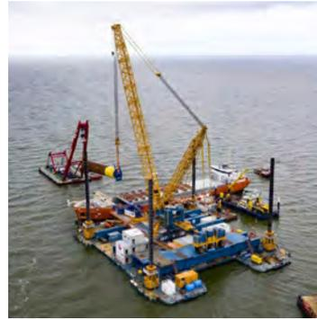
Figure 2. Top view of the CAB on a final tower lake place right before the installation of a monopile.
