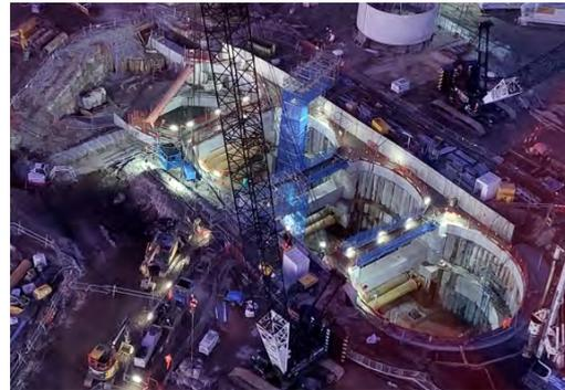
Figure 2. Construction of the Launch chamber.
