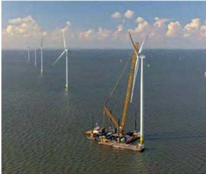
Figure 1. Top view of the CAB with the long boom of 126m during the installation of the blades.
