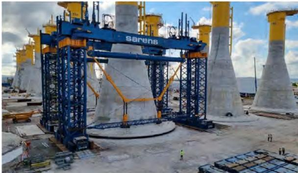
Figure 1. View of the lifting gantry ready to lift a GBS.
