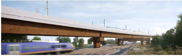
Figure 1. Duddeston Junction Viaduct over existing railway lines – Steel piers/portals - Render.
