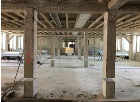
Figure 1. Columns cut during the construction.
