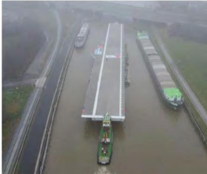
Figure 1. Mobile deck approaching to the lowest canal bridge that had to be crossed.
