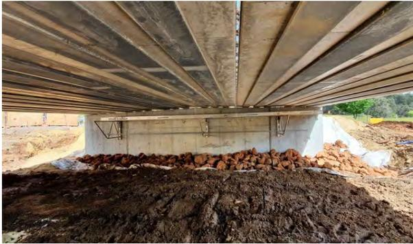
Figure 1. Composite dowel planks installed.
