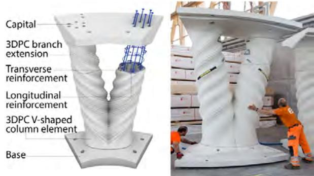
Figure 2. Reinforced 3DPC V-column. Photo and visualisations: A. Anton.
