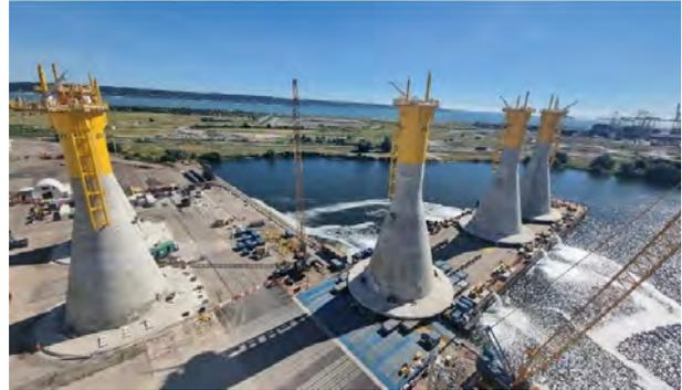
Figure 2. Top view of the last GBS to be loaded out in the cargo barge. External ballasting system in operation.
