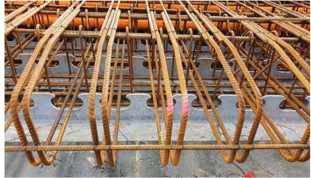
Figure 2. Composite dowel plank reinforcement.
