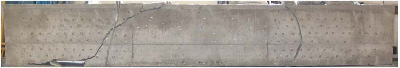
Figure 3. View of specimen after failure.
