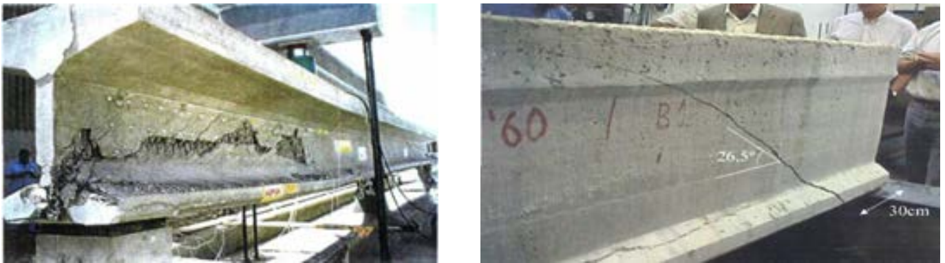
Figure 3. Shear web failures. Left: diagonal tension. Right: by web struts crushing [10].
