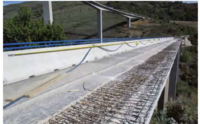
Figure 30. View after radial cutting of the strap
