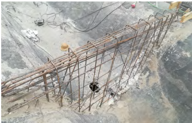
Figure 24. Supporting beam demolition and original underlying rebar configuration.
