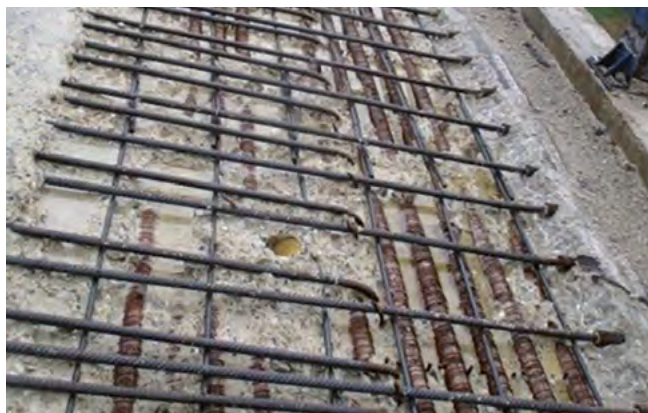
Figure 24. Existing and exposed post-tensioned sheaths.
