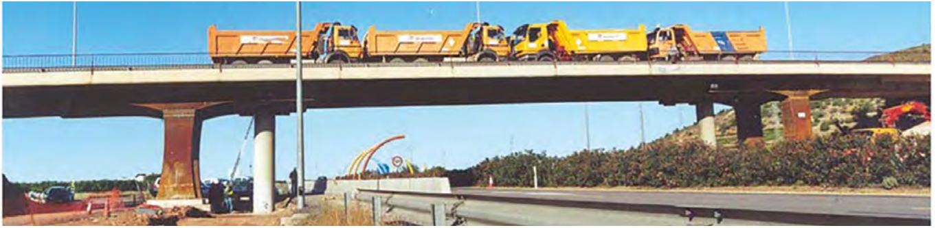
Figure 10. Overpass span enlargement load test.
