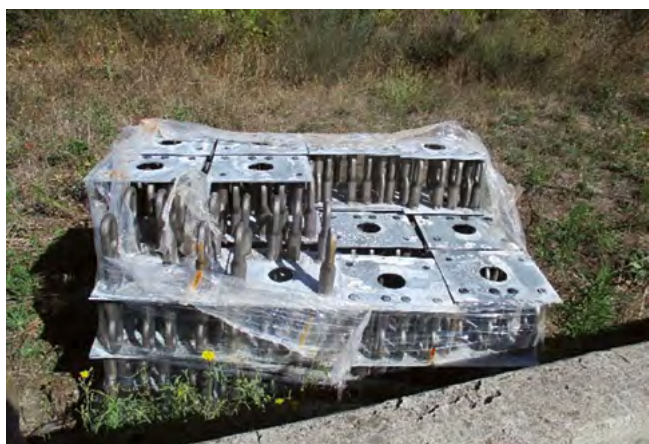
Figure 35. Anchorage of the parapet.
