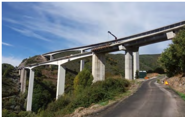
Figure 34. Overview of traveler positioning.
