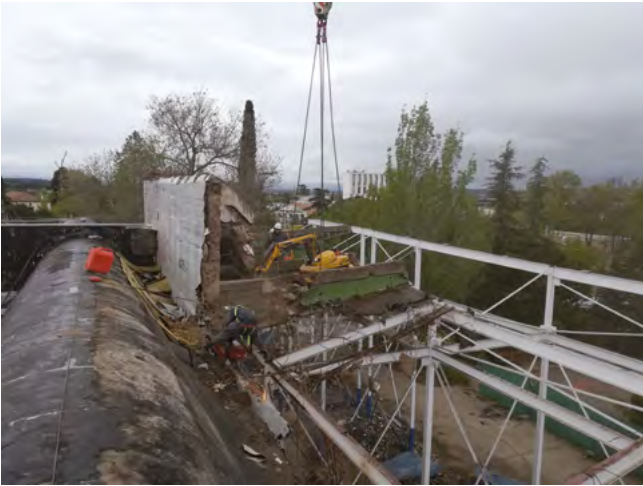
Figure 40. Existing structure demolition.
