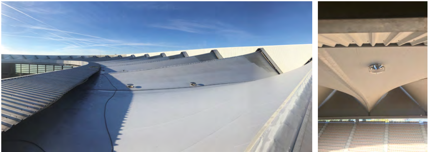
Figure 8. Drainages holes. Credit: schlaich bergemann partner.
