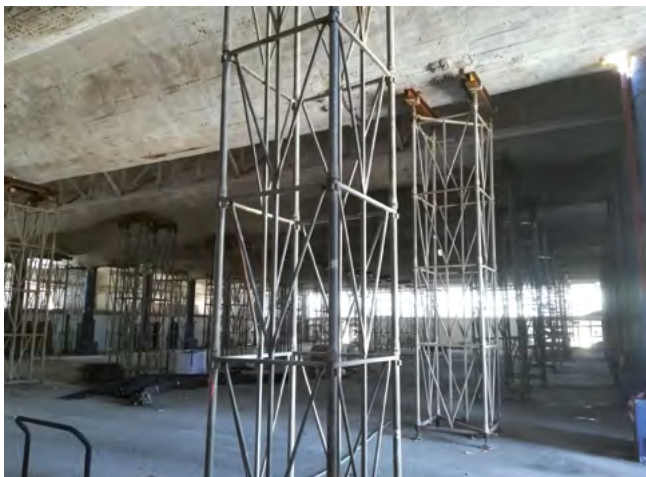
Figure 21. Temporary shoring to ground.
