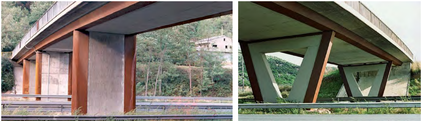
Figure 1. First overpass span enlargements in AP-7 highway (Section: El Vendrel - Salou). 1997. Typological variations.
