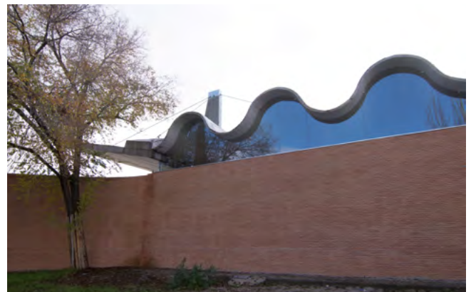
Figure 44. Final appearance of structure and pier top from north façade.
