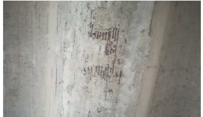
Figure 17a & b. Rebar survey from existing shell roof.
