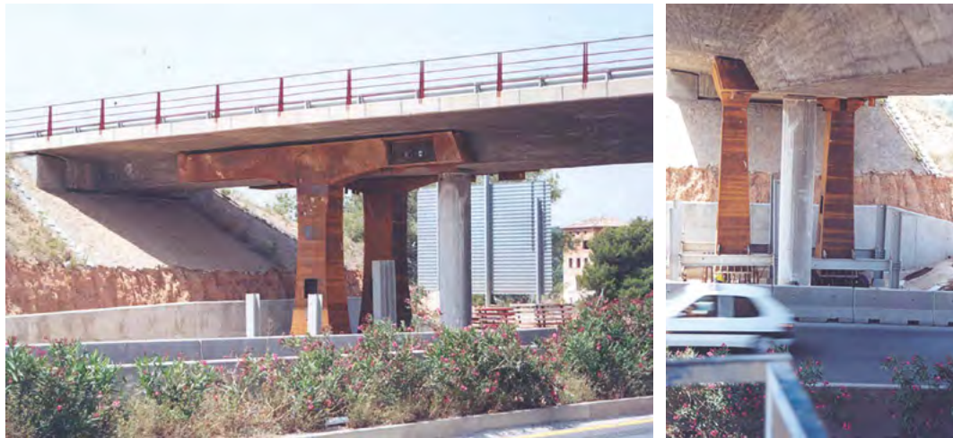
Figure 8. Steel lintel-shaft after transfer operation of dead load.
