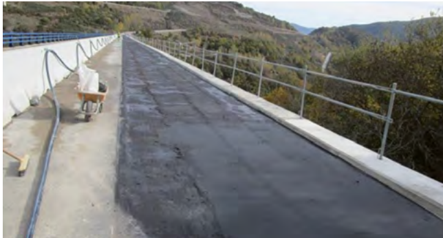
Figure 39. Rebuilt waterproof deck view.
