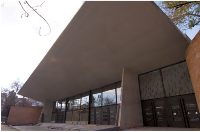
Figure 45. Final appearance of canopy structure.
