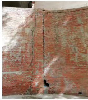
Figure 48. South masonry façade detail between different structural modules.
