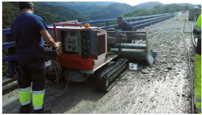
Figure 20. Hydrodemolition Robot.
