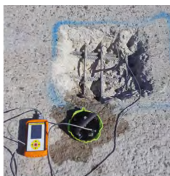
On-site corrosion rate meter
