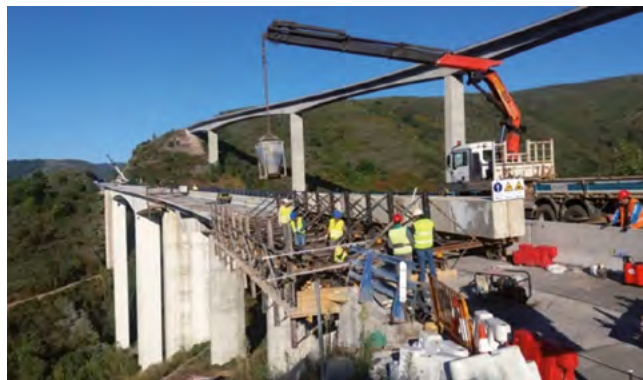
Figure 37. View of the concreting process of the deck and the strap.
