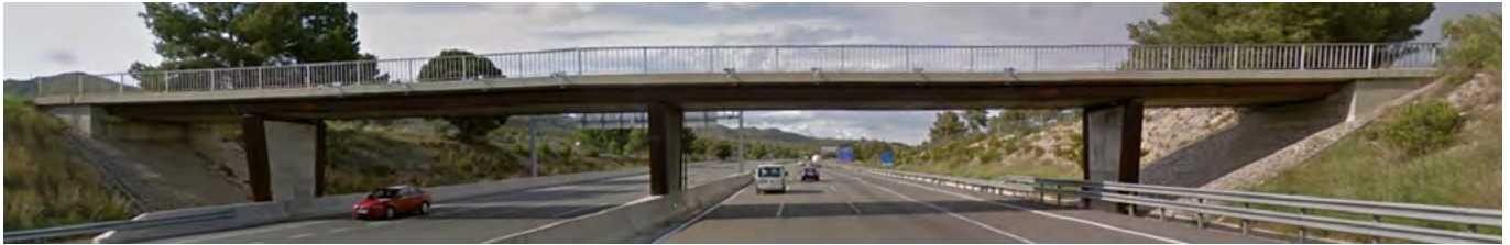
Figure 11. Overpass on the AP-7 highway near El Vendrell.
