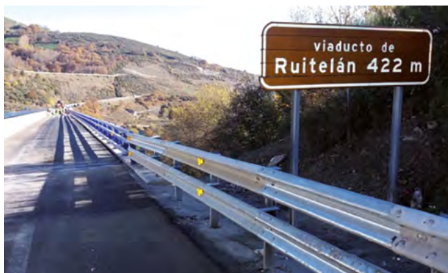
Figure 47. View from Galicia Side Abutment.
