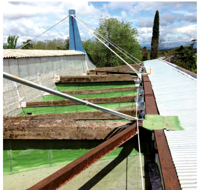
Figure 4. Shoring structure for the pavilion entry canopy.
