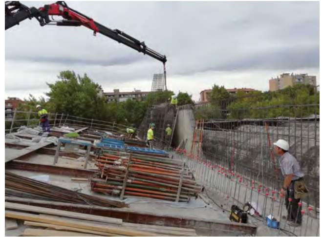
Figure 41. Box girder concreting and joint.
