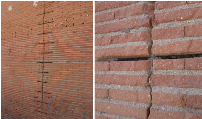
Figure 50. Glass fibre reinforcing for brick walls.
