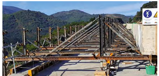
Figure 32. View of the formwork traveler.
