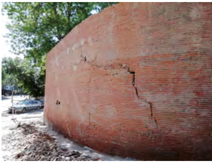
Figure 47. Masonry front wall appearance after plaster removal.
