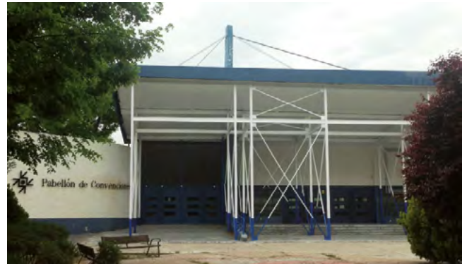
Figure 4. Shoring structure for the pavilion entry canopy.
