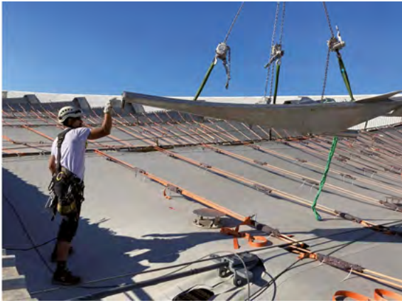
Figure 16. Radial drainage pipes and funnels at Tension Ring installation. Credit: Pfeifer Seil- und Hebetechnik GmbH.
