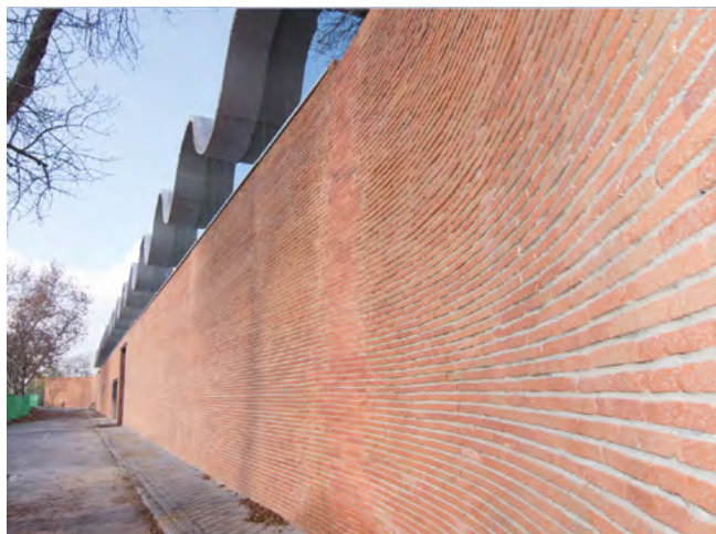
Figure 52. Final appearance of brick walls after rehabilitation.
