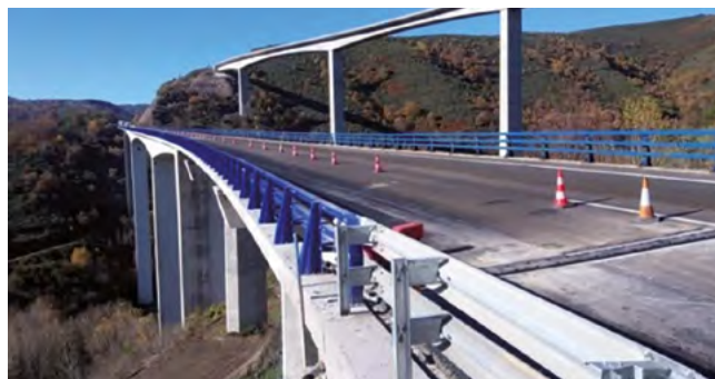
Figure 44. Traffic deviation view.
