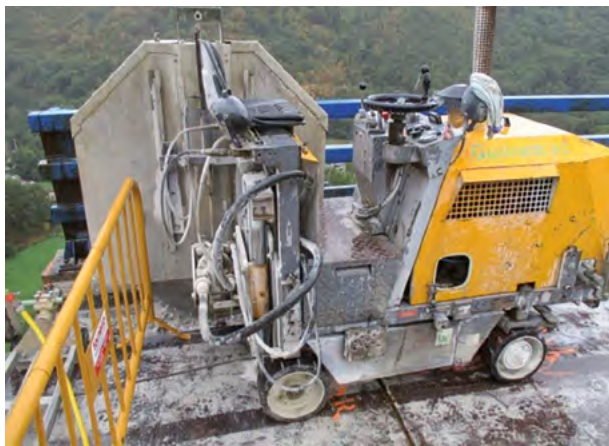
Figure 28 Radial Cutting Machinery.
