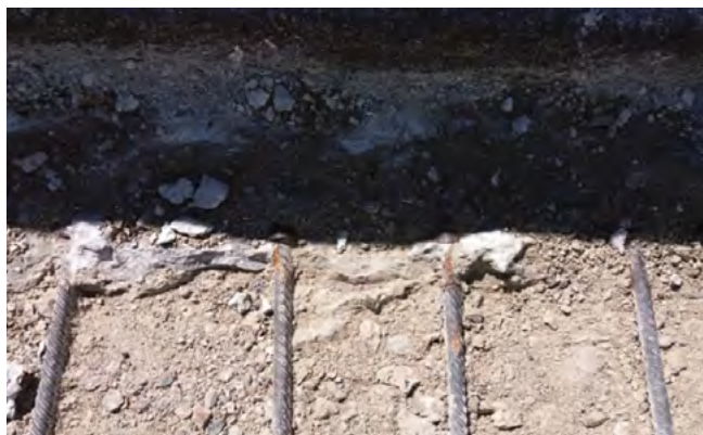
Figure 23. Detail of mechanical couplers.
