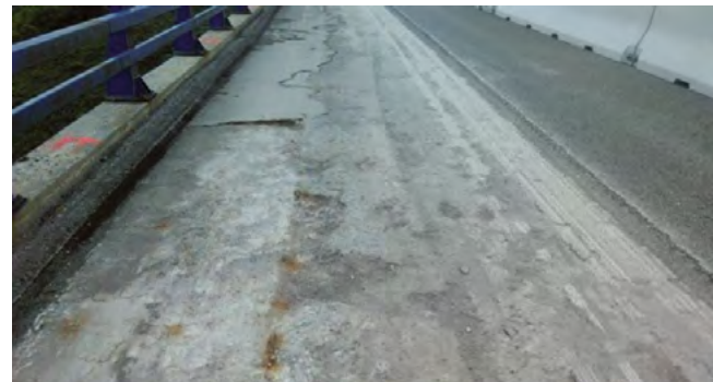
Figure 18. Milling the pavement.
