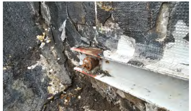
Figure 10. Strengthening cables anchorage on supporting beam.
