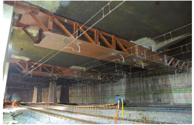
Figure 16. Composite trusses to support removal in Sants Railway Station in Barcelona.
