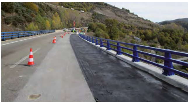
Figure 40. View of the newly installed parapet.
