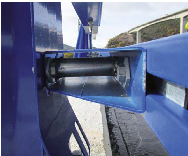
Figure 41. Detail of fixing of the new installed parapet.
