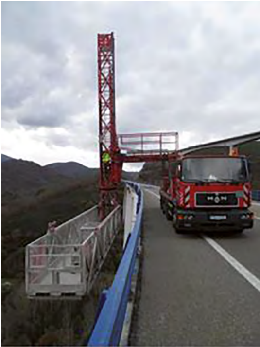
Figure 3. Walkway used in detail inspection.
