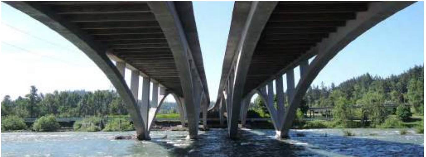
Figure 30. Willamette River Bridge.
