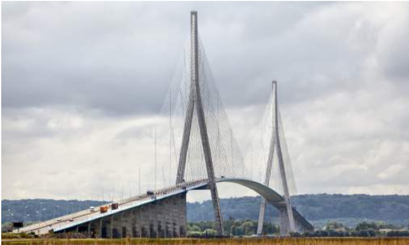
Figure 11. Normandy Bridge, France.
