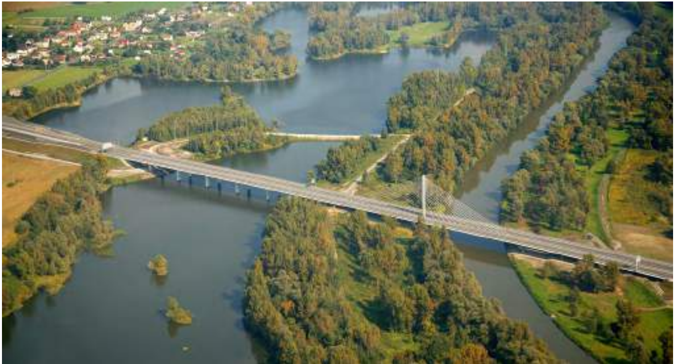
Figure 18. Bridge across the Odra River.
