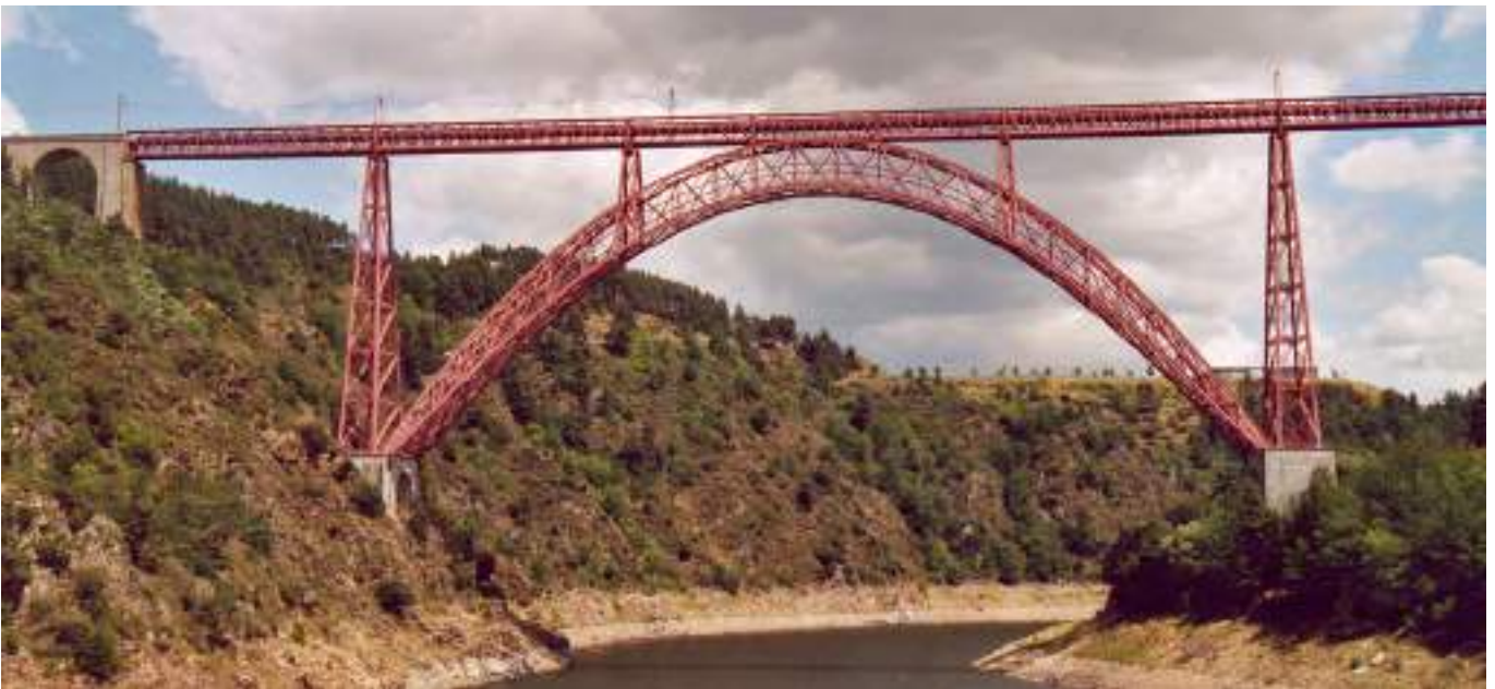
Figure 3. Viaduct of Garabit – 165 m.
