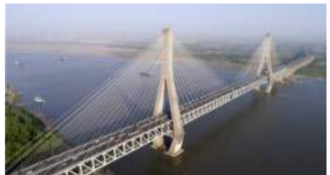
Figure 18. Tiangxingzhou Bridge, Wuhan, China.
