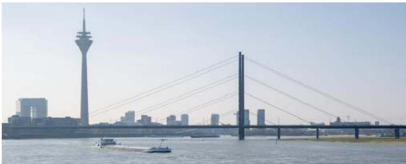
Figure 3. Oberkassel Bridge, Dusseldorf, Germany.
