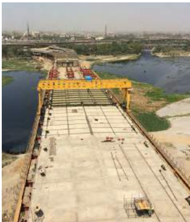
Figure 7. Deck erection with precast elements (left) and in-situ joints between precast elements and steel girder (right). ©schlaich bergemann partner
