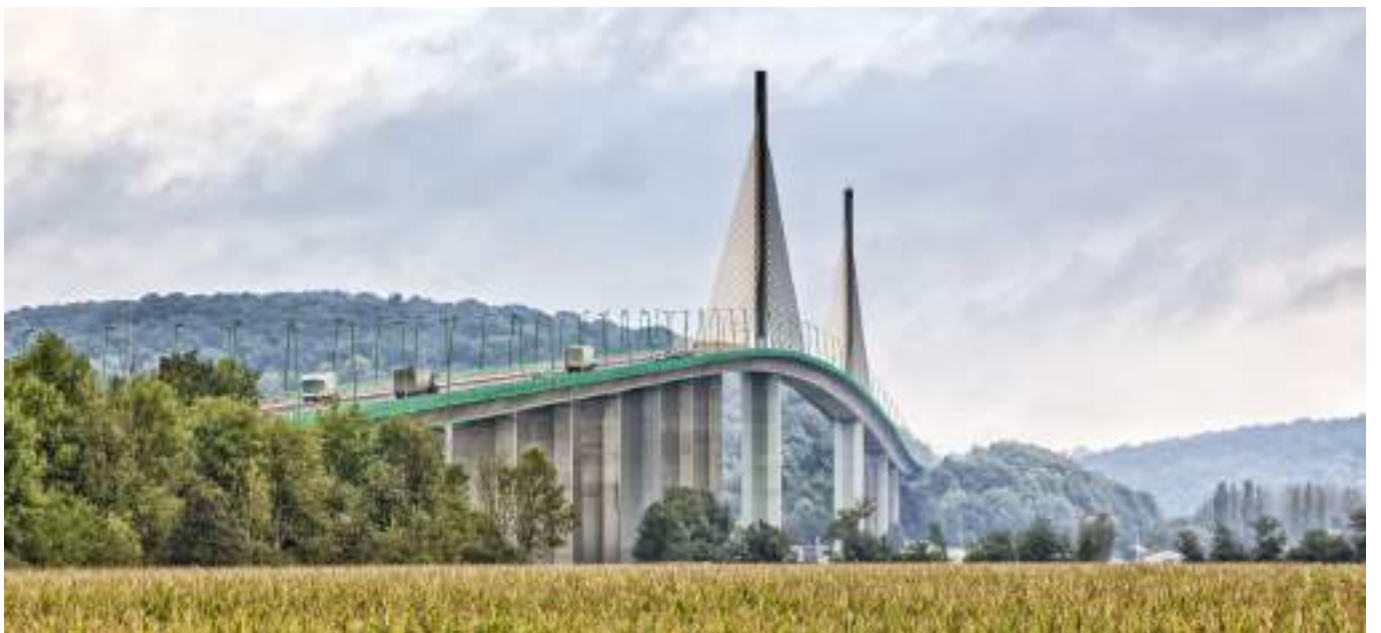
Figure 6. Brottonne Bridge, France.
