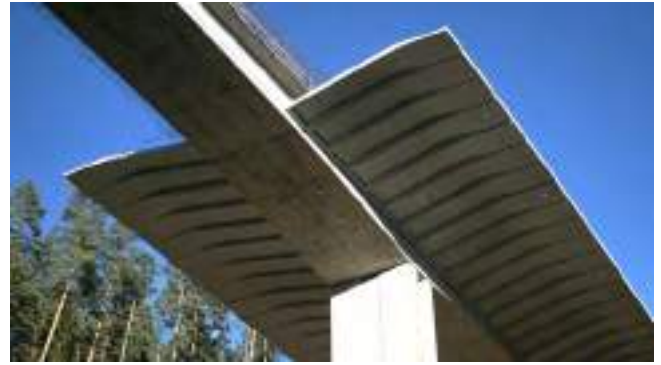
Figure 5. Precast struts - Bridge across the Lodina Creek Valley.
