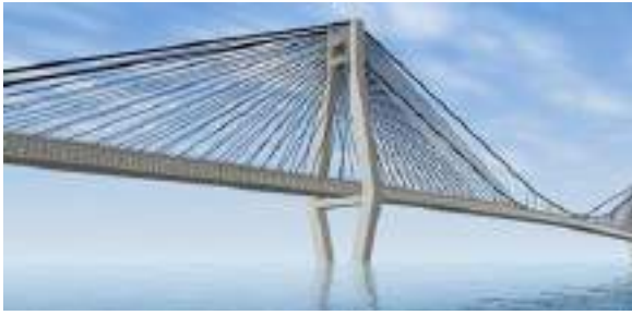
Figure 34. 800m span hybrid bridge
