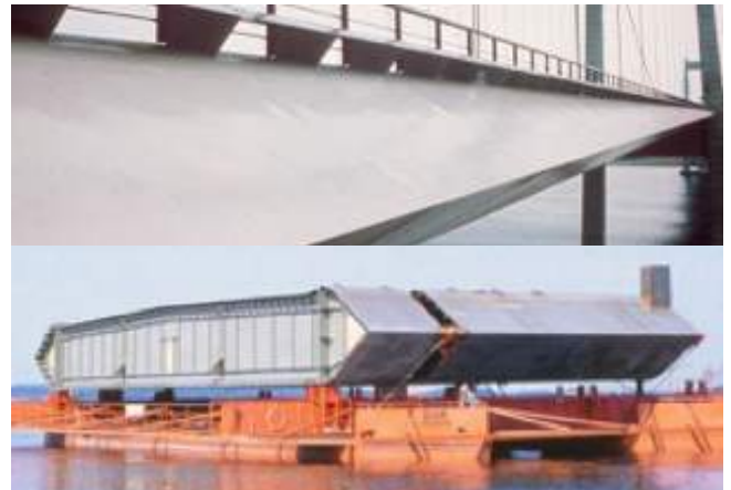
Figure 6. The aerodynamic box girder with wind deflectors.
