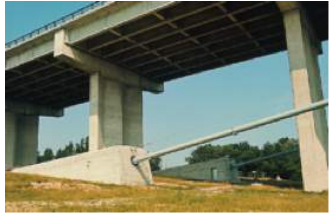
Figure 8. Little Belt Buried Anchorage slab structure.
