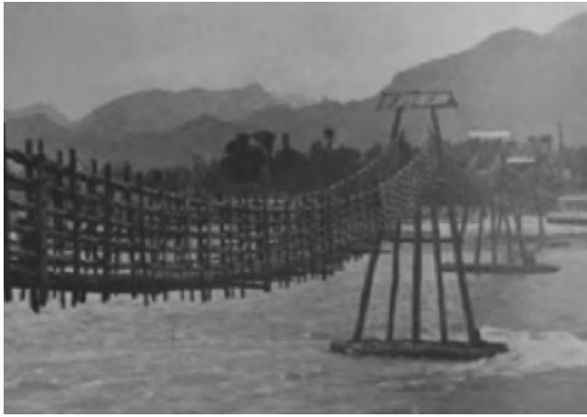
Figure 1. Bamboo Suspension Bridge - Min River - China.
