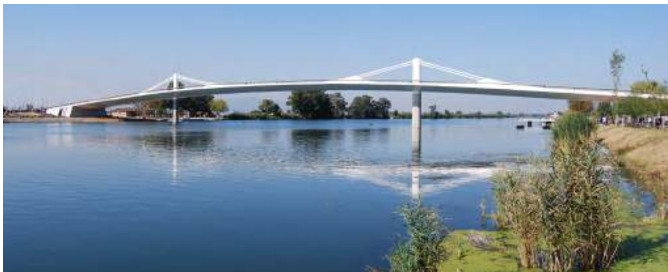
Figure 23. Bridge across the River Ebro.
