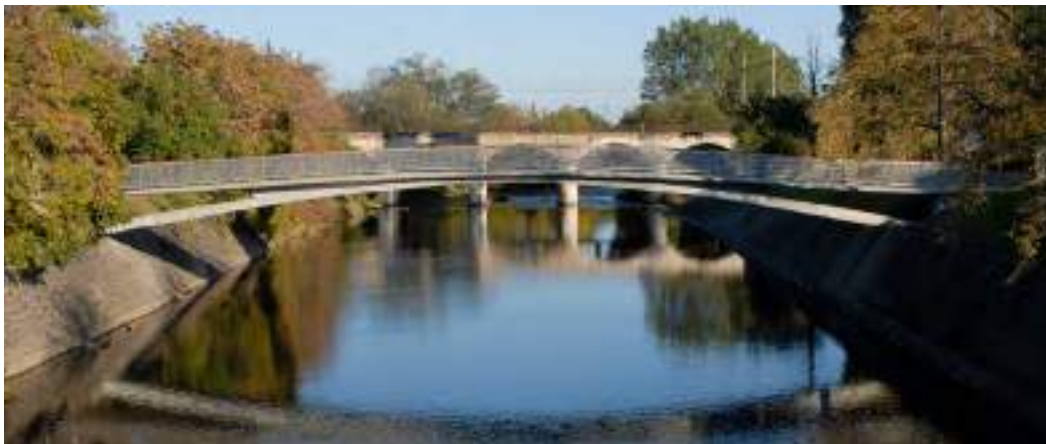
Figure 35. Svratka River Pedestrian Bridge.
