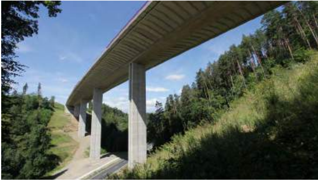
Figure 2. Bridge across the Lodina Creek Valley.
