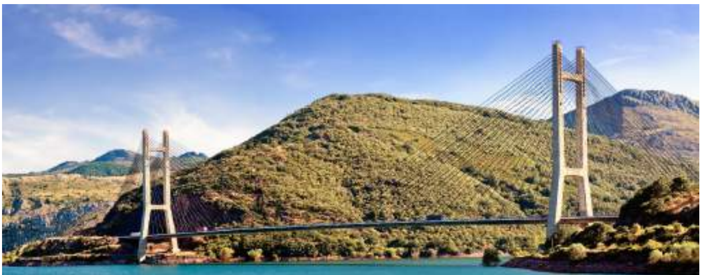
Figure 7. Barrios de Luna Bridge, Spain
