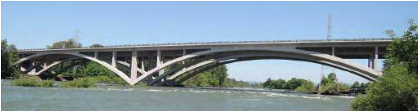
Figure 29. Willamette River Bridge.
