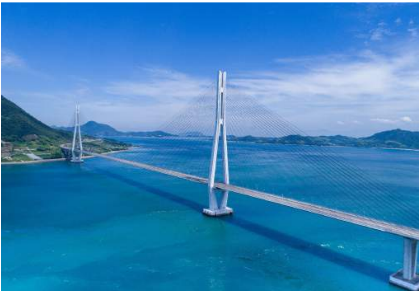
Figure 12. Tatara Bridge, Japan.
