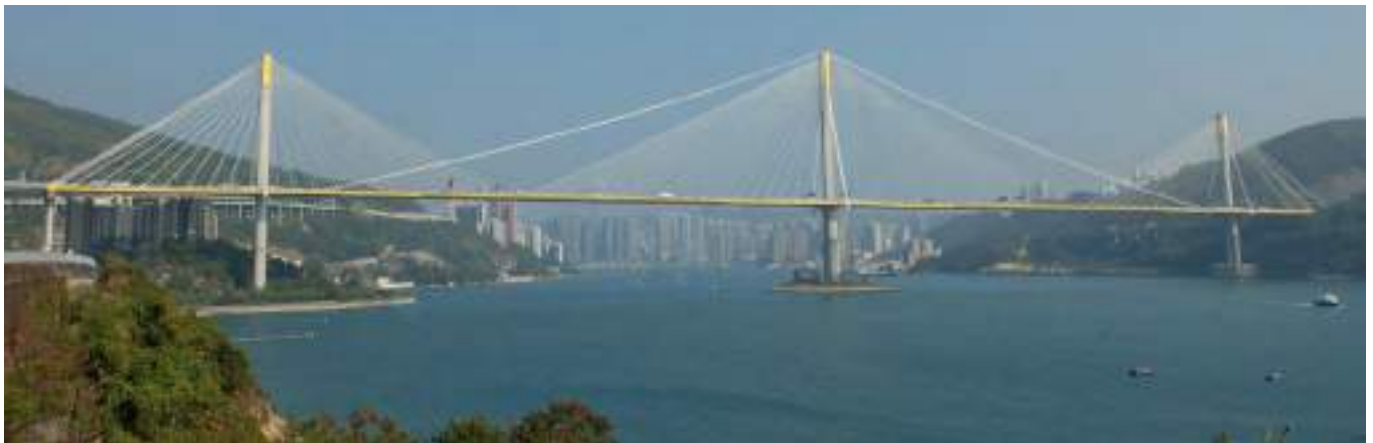
Figure 3. Ting Kau Bridge, Hong Kong. ©schlaich bergemann partner
