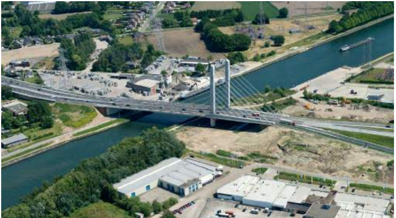
Figure 5. Bridge K03 over Albert Canal, Belgium. ©Jan de NUI, Patrick Henderyckx
