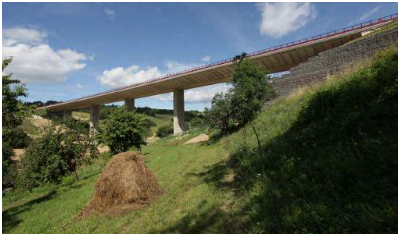
Figure 1. Bridge across the Lazny Creek Valley.
