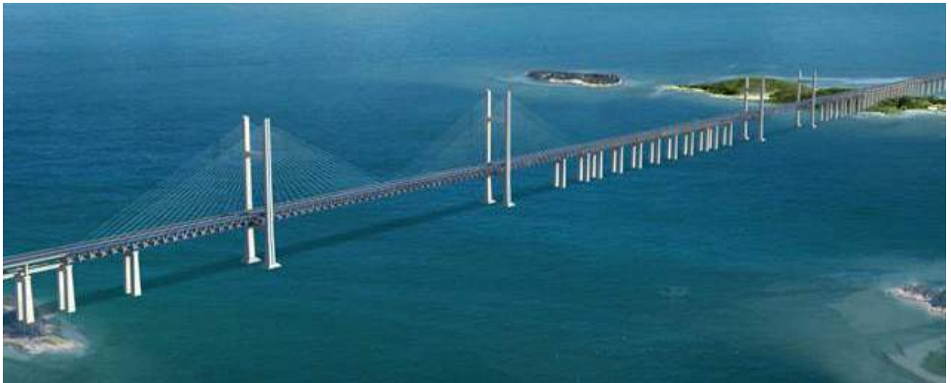
Figure 19. Pintan Strait Crossing, Fujian, China.
