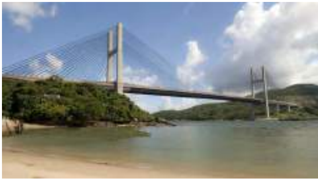
Figure 13. Kap Shui Mun Bridge, Hong Kong.
