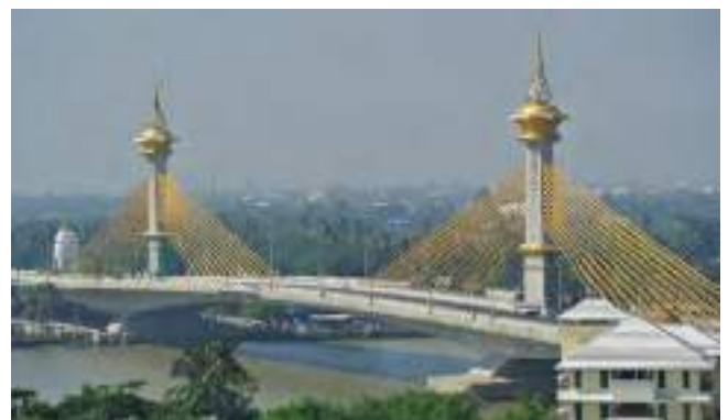
Figure 15. Nonthaburi Bridge (Thailand)
