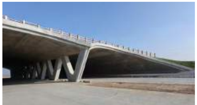
Figure 28. Wildlife Overpasses, Czech Republic.
