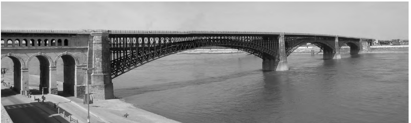
Figure 5. Eads Bridge (1874) – 3 x 158,5 m.
