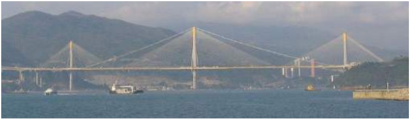
Figure 23. Ting Kau Bridge, Hong Kong.
