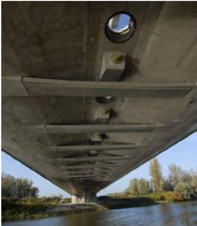
Figure 20. Deck of the suspended spans - Bridge across the Odra River.
