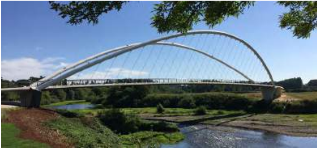
Figure 34. Minto Island Pedestrian Bridge.
