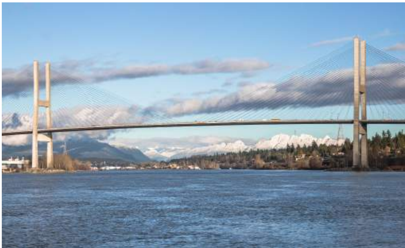
Figure 8. Alex Fraser Bridge, Vancouver, Canada.
