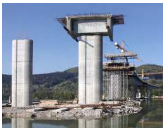
Figure 16. Deck of the approach spans of the Bridge across the River Vah's Reservoir.
