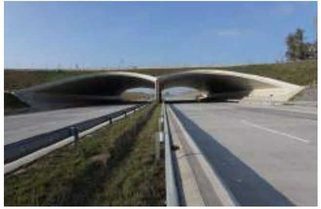
Figure 27. Wildlife Overpasses, Czech Republic.
