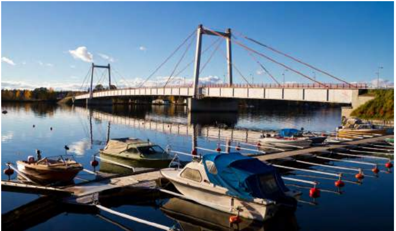
Figure 1. Stromsund Bridge, Sweden.
