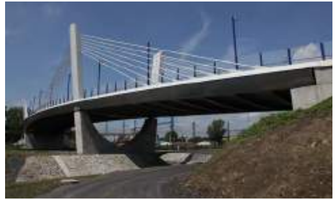
Figure 21. Bridge across the Railway Station at Bohumin.
