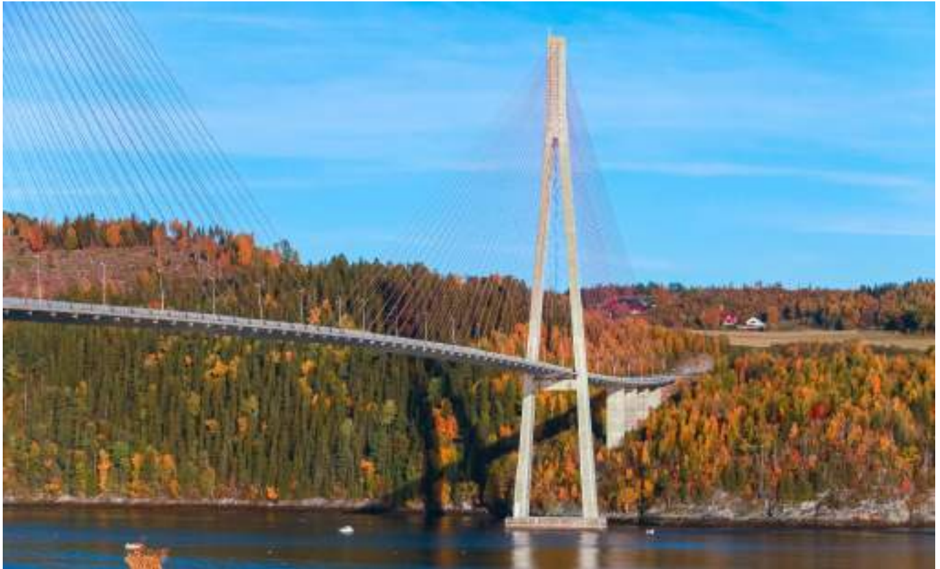
Figure 9. Skarsundet Bridge, Trondheim, Norway.
