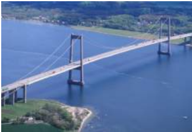
Figure 5. The Little Belt Bridge, Denmark.
