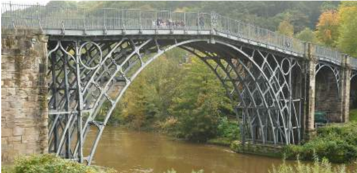
Figure 1. Iron bridge – 60 m.
