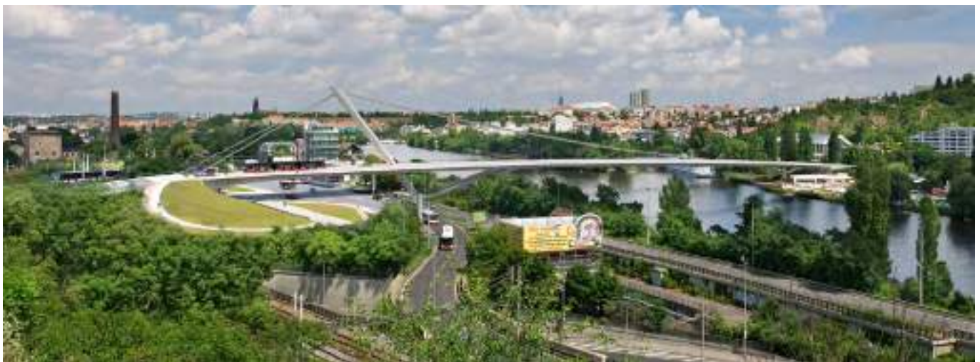
Figure 20. Dvorecky bridge. (FHECOR).
