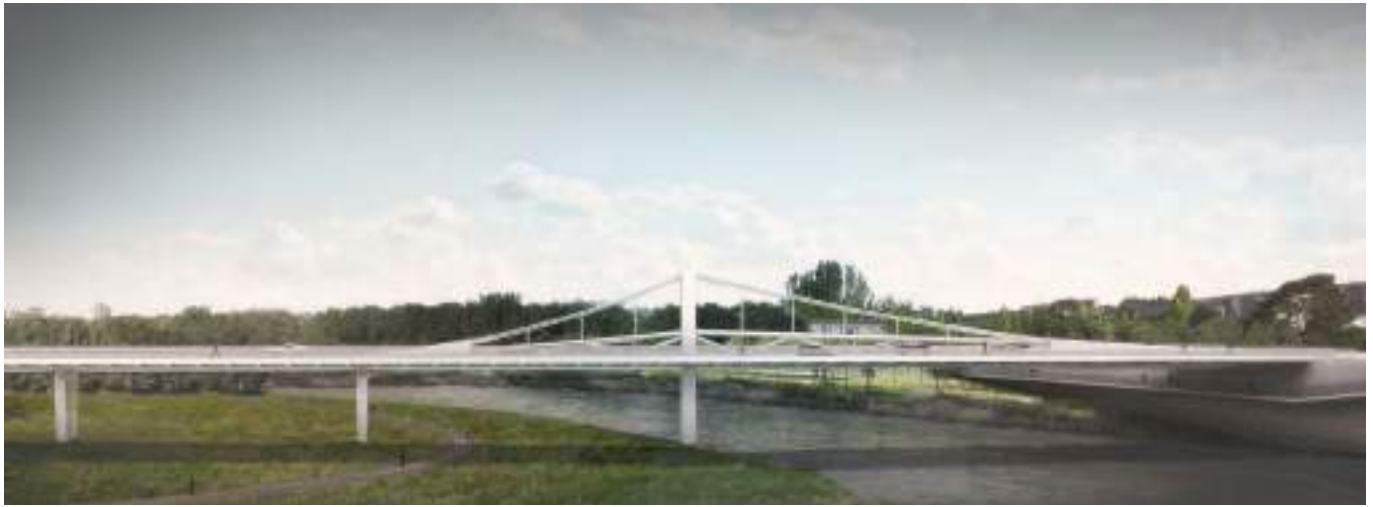
Figure 19. Arga bridge. (FHECOR).
