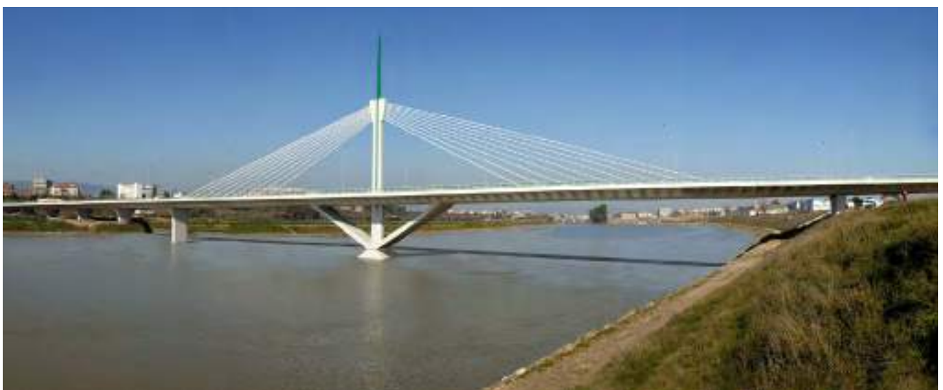
Figure 12. Andalusia Bridge (Córdoba) J. Manterola. Source: Carlos Fernández Casado S.L.
