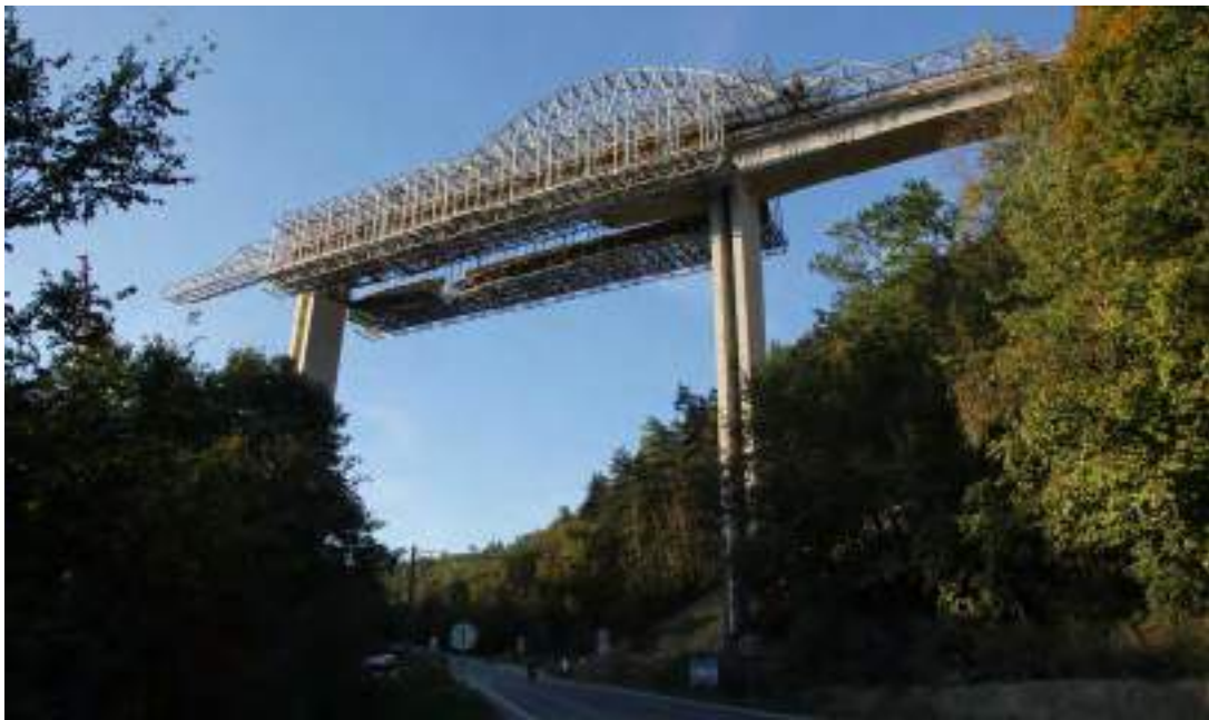
Figure 3. Movable scaffolding - Bridge across the Lodina Creek Valley.
