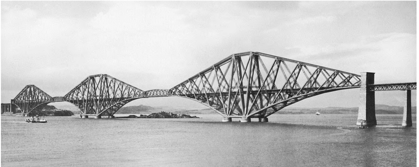
Figure 4. Firth of Forth bridge (1890) – 2 x 521 m.
