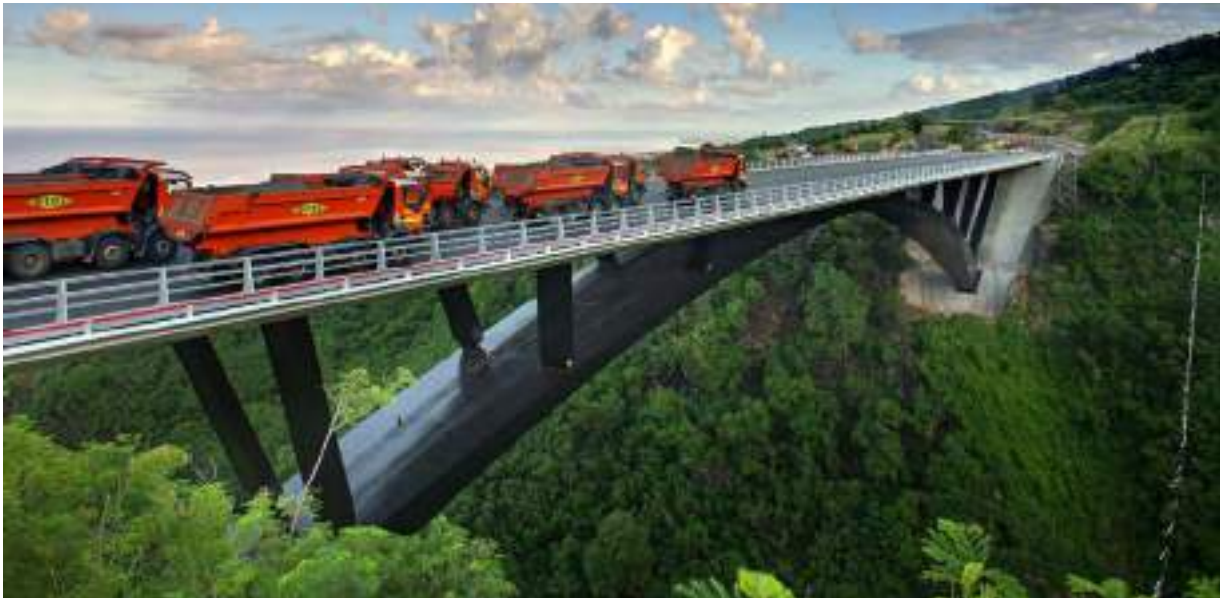
Figure 23. Arch bridge over the Ravine Fontaine.
