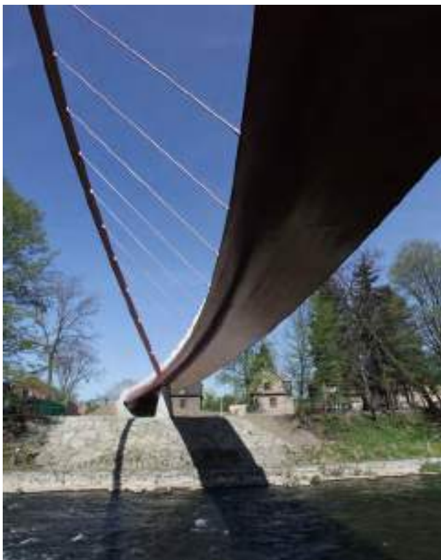
Figure 31. Pedestrian Bridge across the Olse River.
