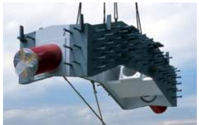
Figure 10. Separated steel box anchorage
