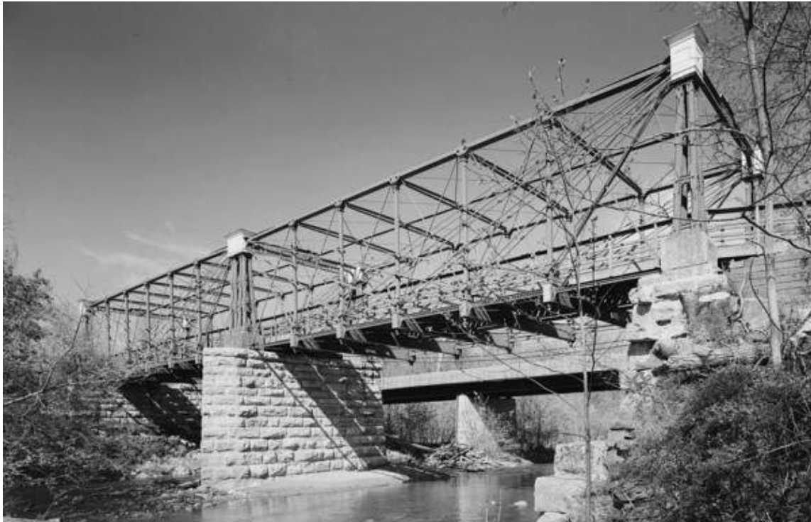
Figure 2. Early hybrid structures XIXth Century. Source: Structurae. Image-ID: 6316.
