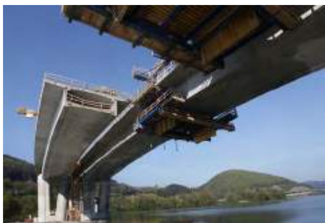
Figure 15. Deck of the main spans of the Bridge across the River Vah's Reservoir.
