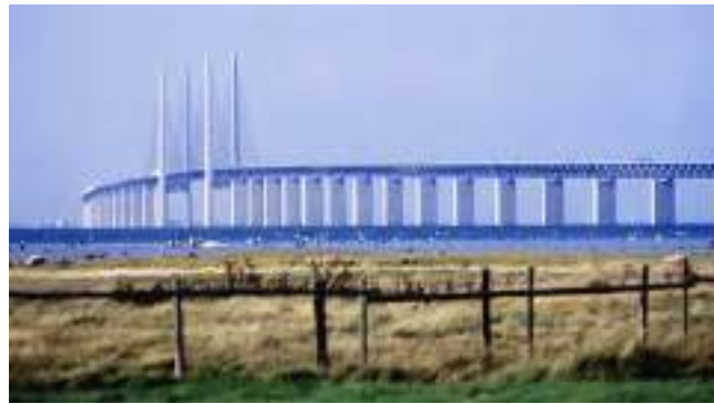
Figure 14. Oresund Crossing, Denmark & Sweden.
