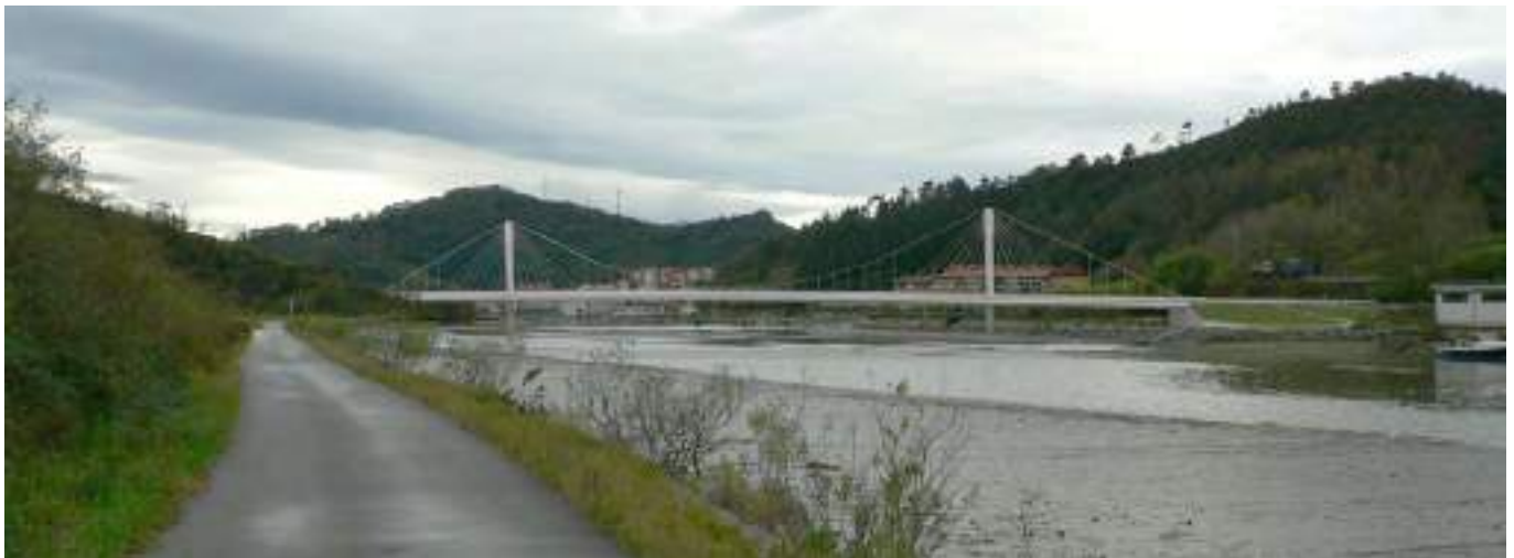
Figure 7. Orio Bridge. (FHECOR).
