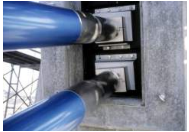
Figure 2. Saddle anchorage of extradosed cables
