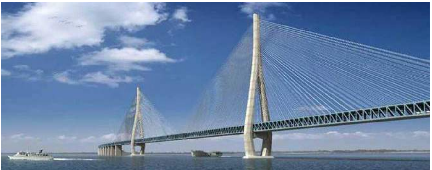
Figure 20. Hutong Bridge, Shanghai, China.
