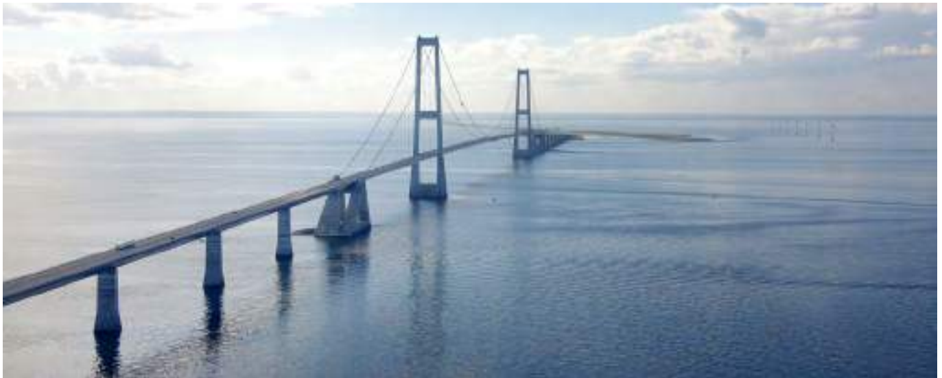
Figure 13. Great belt Suspension Bridge - 1,624 m main span.
