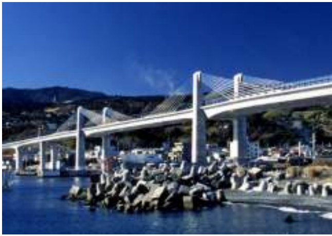
Figure 1. Odawara Blueway Bridge
