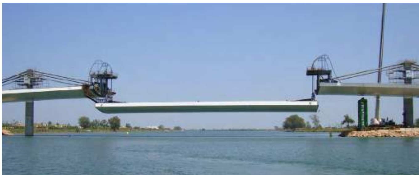
Figure 24. Lifting of the deck of the Bridge across the River Ebro.
