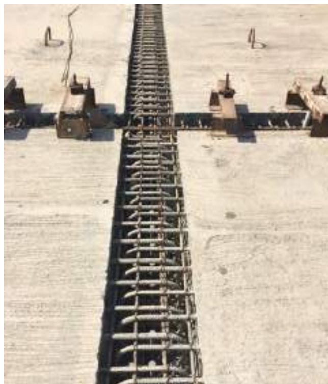
Figure 7. Deck erection with precast elements (left) and in-situ joints between precast elements and steel girder (right). ©schlaich bergemann partner
