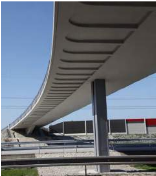
Figure 26. Deck of the Pedestrian Bridge across the motorway D1.
