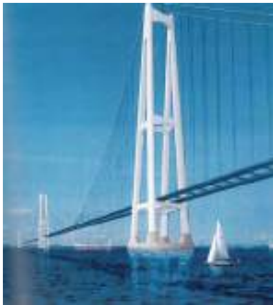
Figure 17. Gibraltar Strait - 3 x 3500 m suspension bridge solution.
