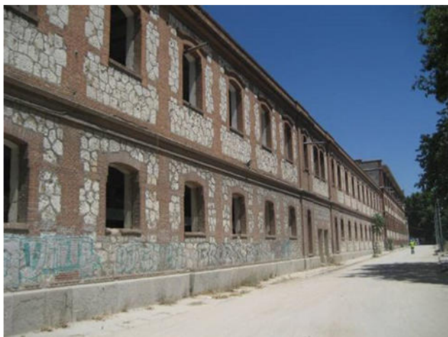
Figure 4. Warehouse 9. Outside view.
