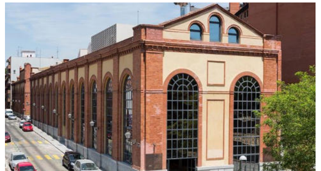
Figure 22. Outside view of the building.
