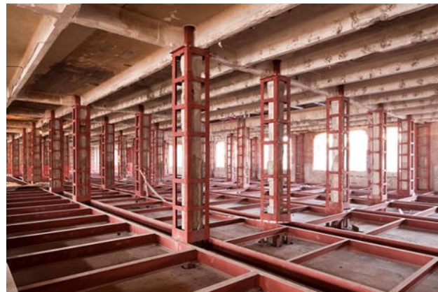
Figure 7. New steel structure in warehouse 8.
