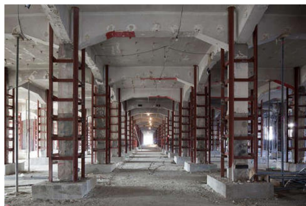
Figure 8. New steel structure in warehouse 9.
