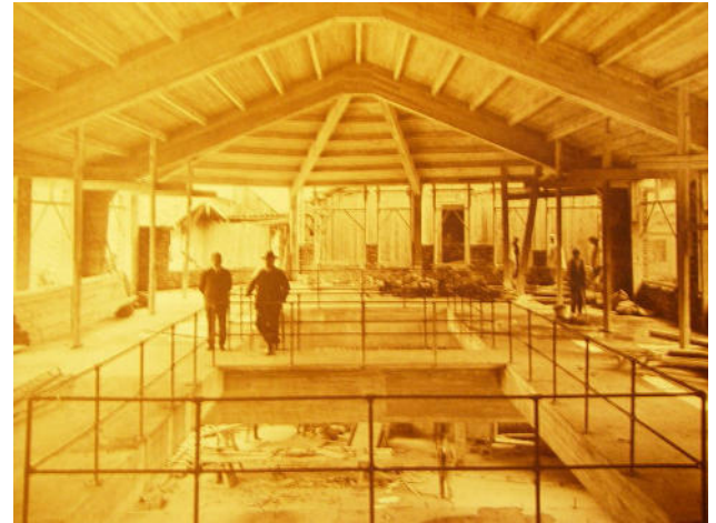
Figure 15. Inside view of the original Serrería.
