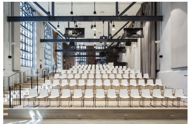
Figure 24. Google Campus Madrid auditorium, featuring the new trusses based on the old beams of the demolished slab floors.
