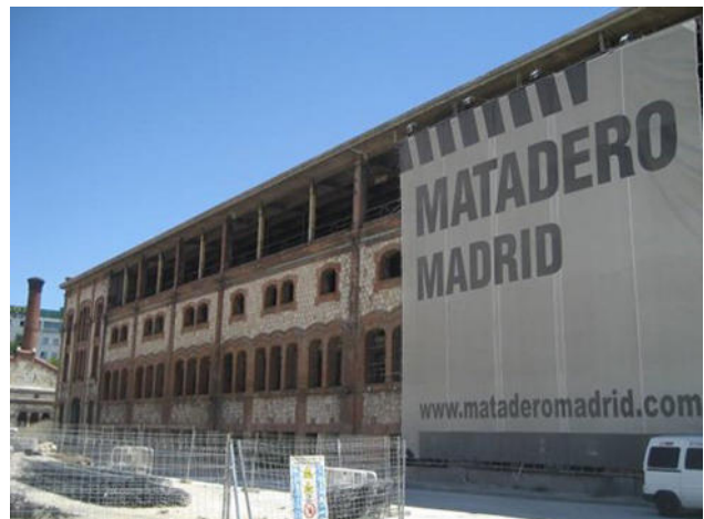
Figure 3. Warehouse 8. Outside view.
