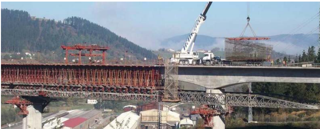
Figure 29. Positioning pre-assembled reinforcement on deck.
