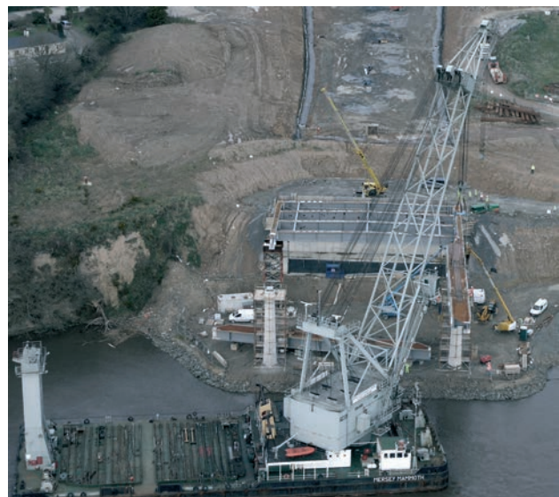
Figura 39. Colocación del tramo de espera mediante grúa flotante Figure 39. Installation of the end span by a floating crane
