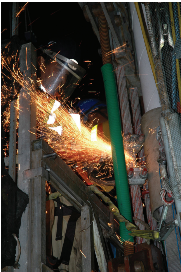
Figura 39. Corte de los cables originales Figure 39. Cutting the original cables
