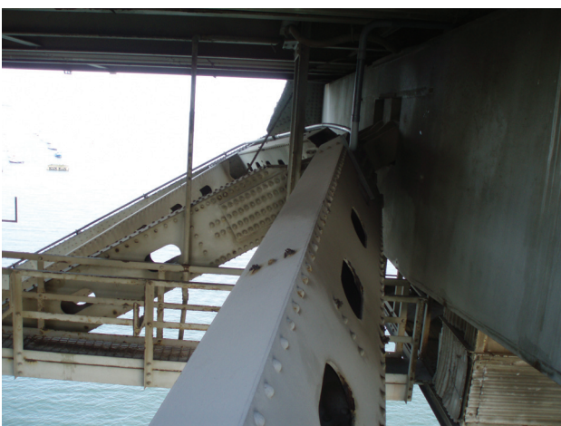
Figura 13. Rótula en plano inferior de celosía Figure 13. Joint on lower truss
