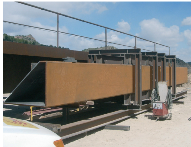
Figura 50. Riostra de voladizo Figure 50. Cantilever brace
