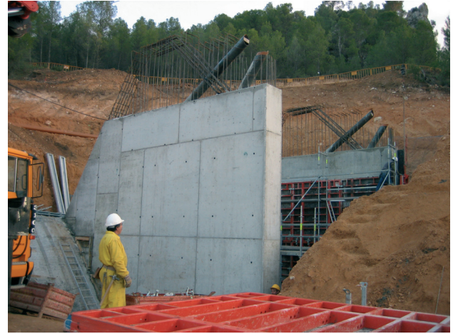
Figura 10. Estribo 2. Vainas de retenida Figure 10. Abutment 2. Guyline sheaths
