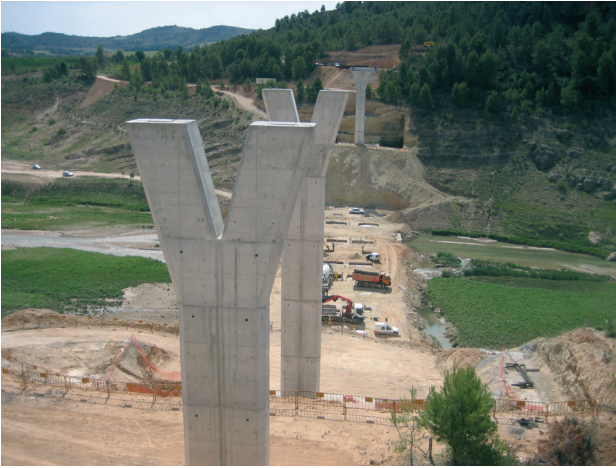
Figura 9. Pilas y plataforma del bowstring Figure 9. Piers and bowstring platform
