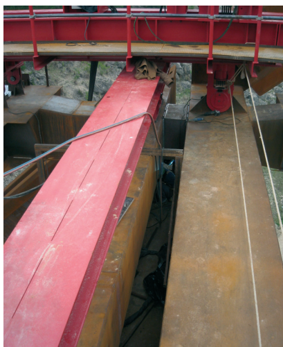
Figura 23. Carrete de unión en tablero Figure 23. Extension plate on deck
