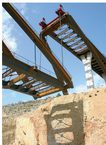
Figura 20. Izado a media carrera Figure 20. Hoisting operation
