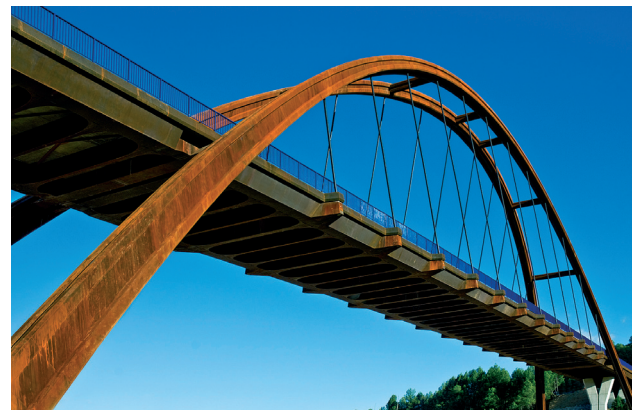
Figura 56. Acabados (II) Figure 56. Finishes (II)
