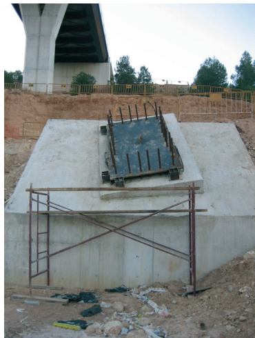
Figura 45. Replanteo placa apoyo Figure 45. Support plate stake-out
