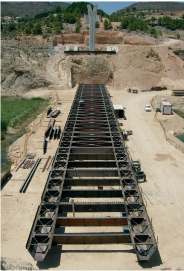
Figura 13. Bowstring (I). Tablero Figure 13. Bowstring (I). Deck
