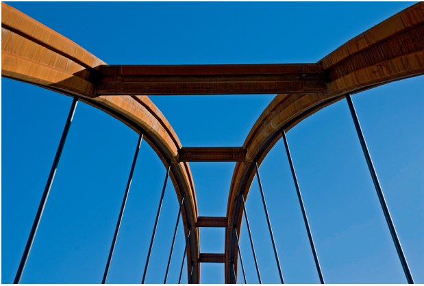
Figura 55. Acabados (I) Figure 55. Finishes (I)
