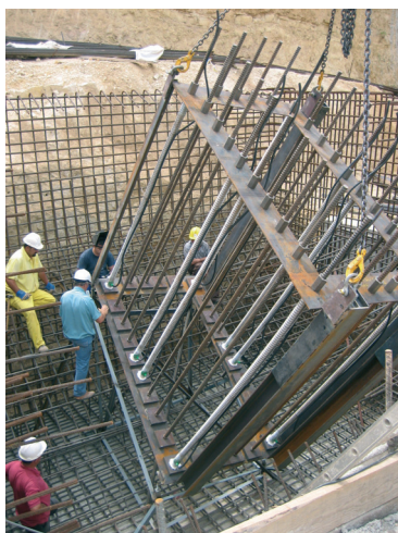
Figura 44. Replanteo de barras Figure 44. Bar stake-out
