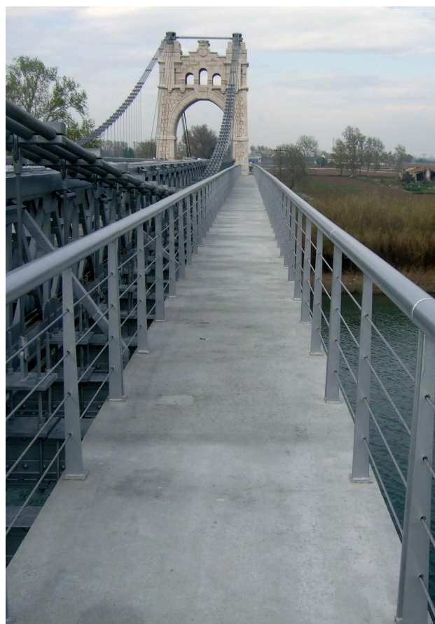
Figura 40. Nueva acera terminada. Figure 40. Finished walkway.
