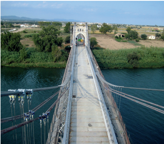
Figura 19. Cables durante la transferencia de cargas del sistema provisional al definitivo. Figure 19. Cables during load transfer from provisional to permanent system.
