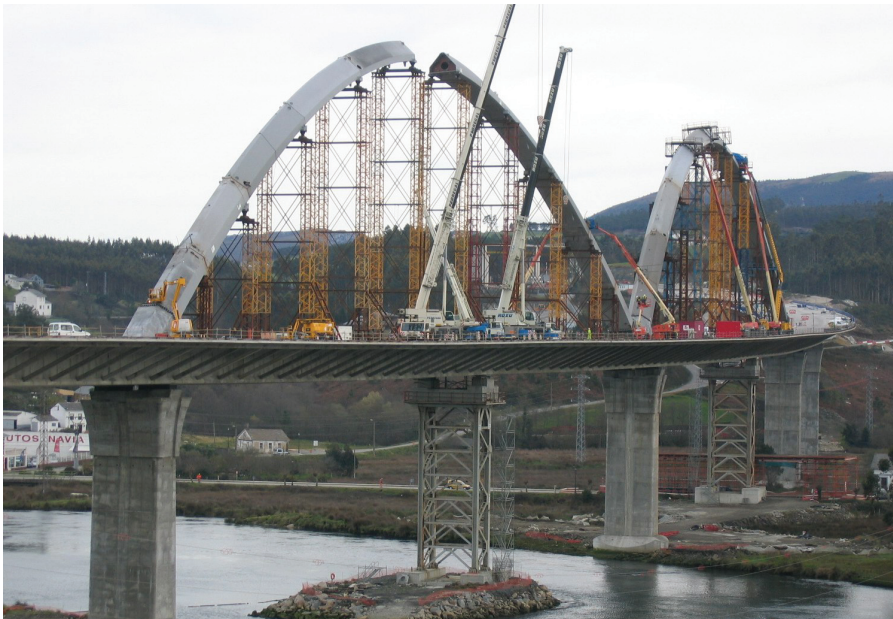
Figura 19. Montaje de arcos. Figure 19. Arch assembly.
