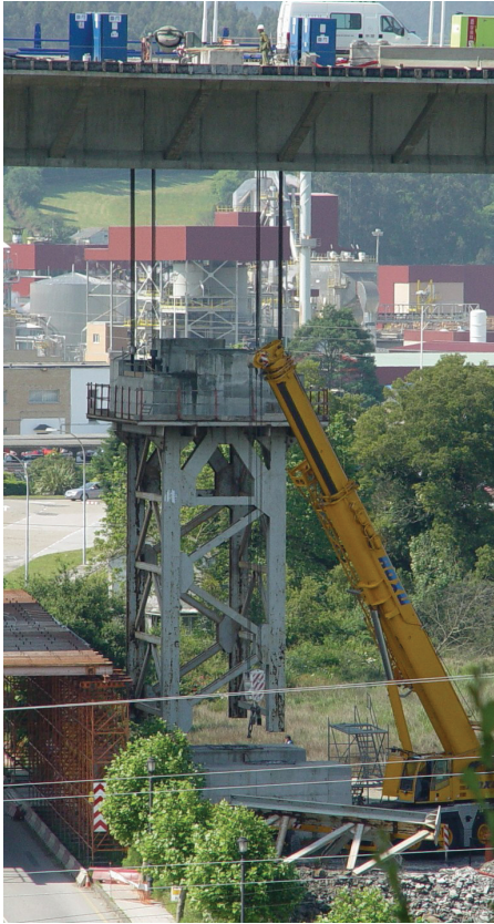
Figura 22. Retirada de pilas provisionales. Figure 22. Removal of provisional piers.
