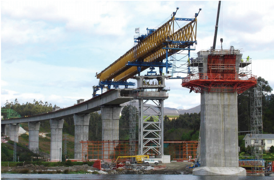
Figura 17. Montaje de dovelas. Figure 17. Segment assembly.
