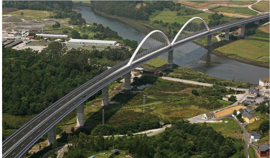
Figura 23. Vista aérea del viaducto acabado. Figure 23. Aerial view of the finished viaduct.
