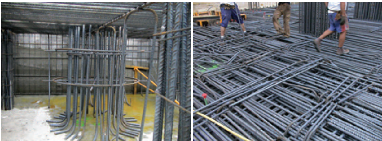
Figura 8. Arranque de soportes de torre y cierre de torretas de cortante. Figure 8. Start of the tower supports and end of the shear turrets.
