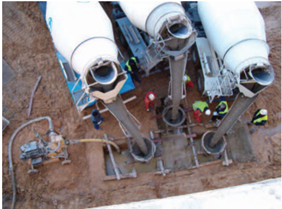
Figura 6. Hormigonado de pantallas con tubo tremi y tres camiones hormigonera. Figure 6. Pouring concrete for the diaphragm walls with tremies and three concrete mixers.
