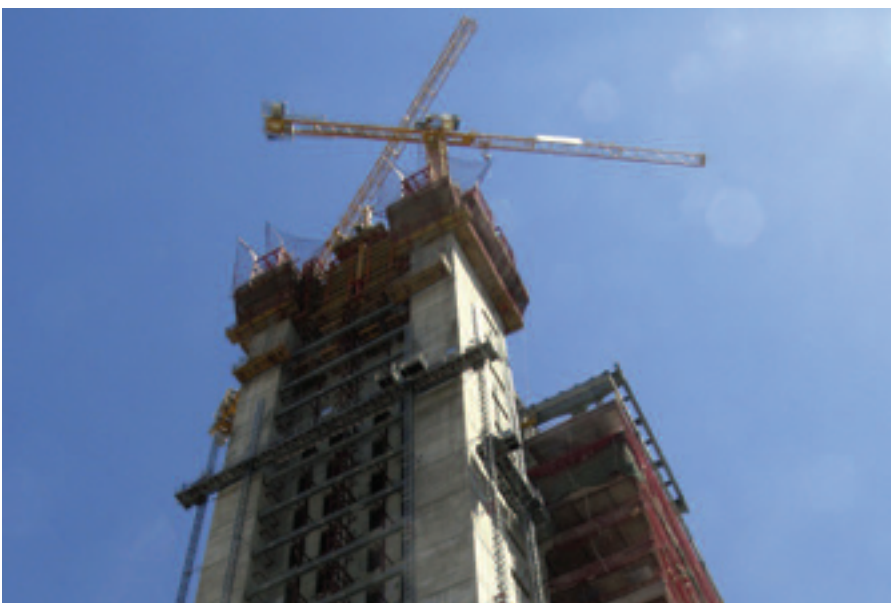
Figura 6. Plataformas eléctricas de fachada. Figure 6. Electrically powered façade platforms.
