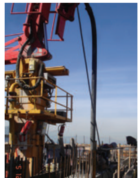
Figura 4. Bombeo de hormigón. Figure 4. Concrete pumping.
