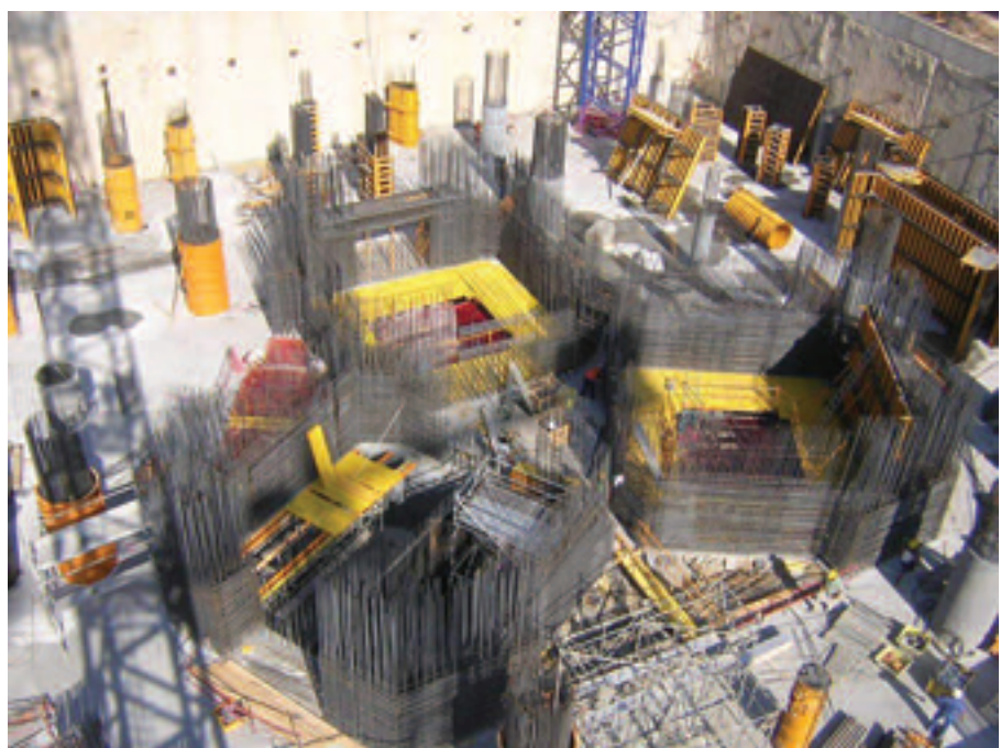
Figura 13. Vista general de armado y encofrado de núcleo y soportes. Figure 13 General view of the reinforcement and formwork of the core and supports
