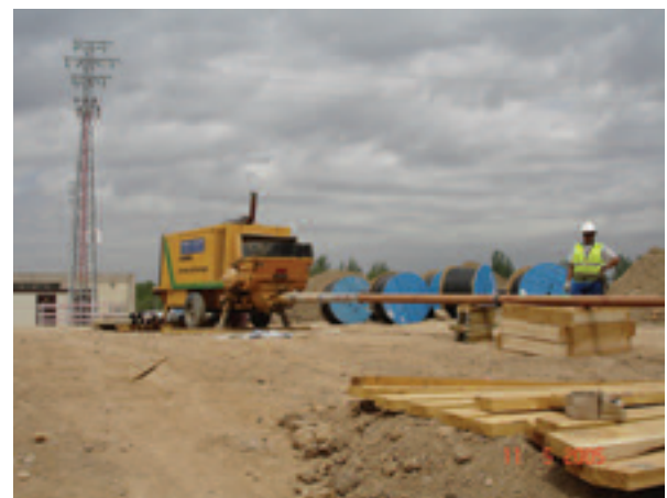
Figura 3. Bombeo de hormigón. Figure 3. Concrete pumping.
