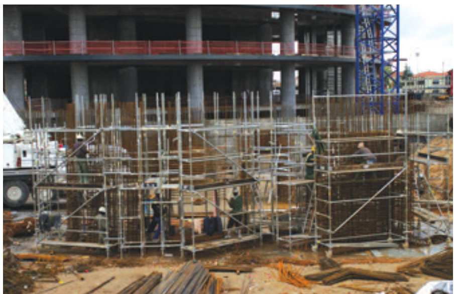
Figura 11. Vista de taller de ferralla con despiece de armado de núcleos. Figure 11. View of the rebar workshop with a breakdown of the core reinforcement.
