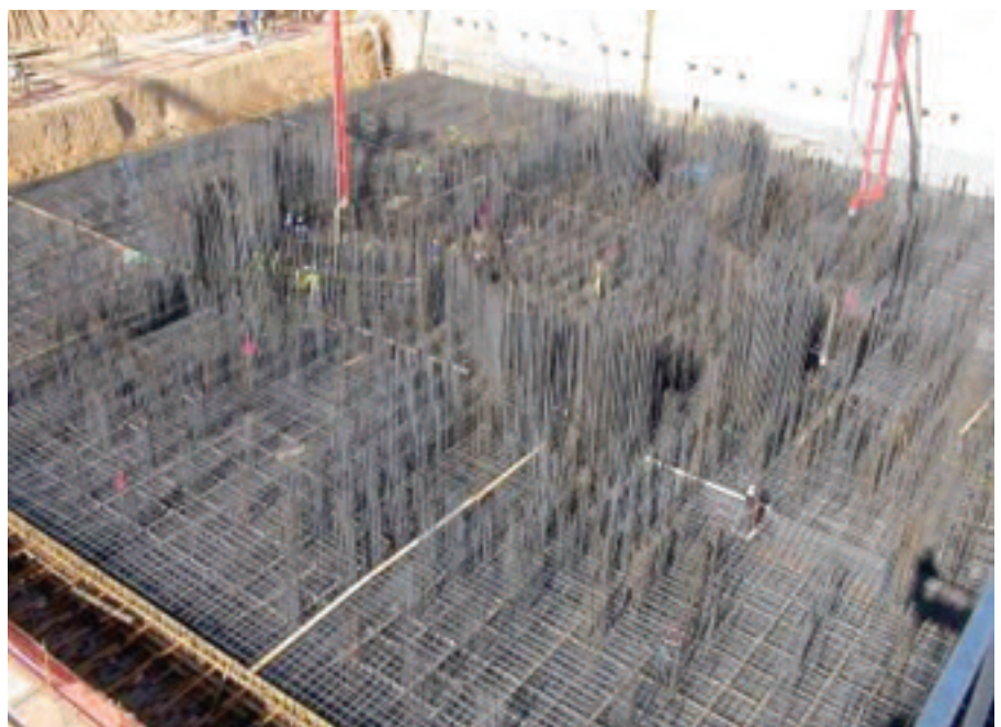
Figura 1. Vista general del ferrallado de la primera tongada. Figure 1. General view of the rebars of the first concrete lift.
