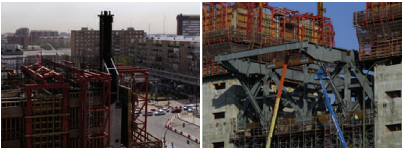
Figura 20. Pilar embebido y cerchas principales. Figure 20. Embedded column and main trusses.
