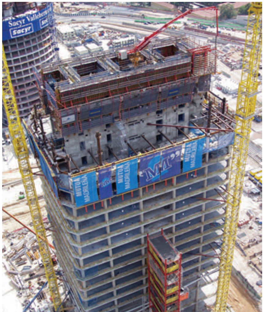
Figura 1. Vista general de grúas y ascensor de obra. Figure 1. General view of cranes and construction hoist.
