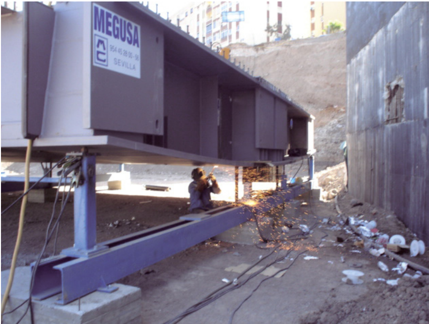
Figura 16. Diafragma de estribo 1. Figure 16. Diaphragm of abutment 1.
