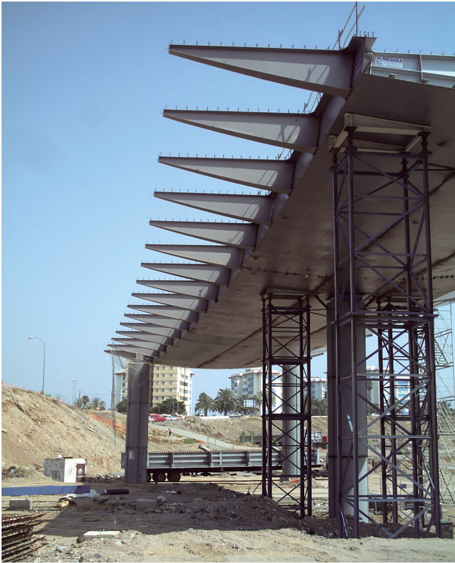
Figura 14. Costillas metálicas Figure 14. Metal ribs.
