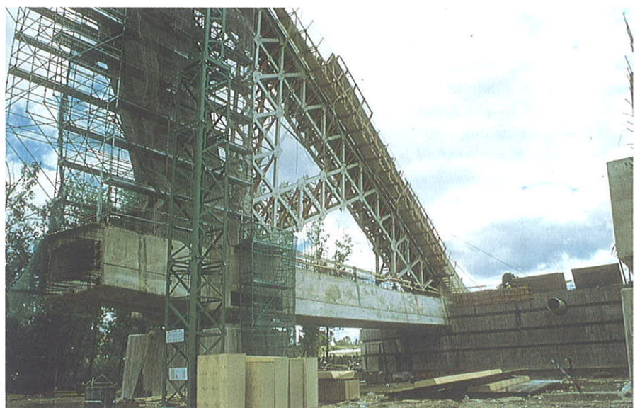
Foto 4. Vista de la cimbra de la vela inclinada. Figure 4. View of the centering used for the construction of the inclined sail.
