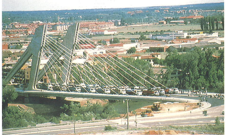
Figura 12. Vista del puente durante la prueba de carga. Figure 12. A view of the bridge during the loading test.
