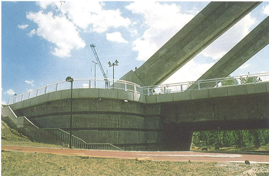
Figura 15. Vista del contrapeso final con los arranques de velas en el puente acabado. Figure 15. View of the final block of counterweight with the beginning of the inclined sails.
