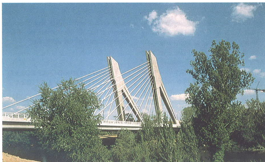
Figura 9. el puente acabado desde la margen del río. Figure 9. The finished bridge seen from the margin of the river.
