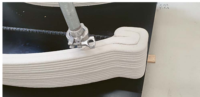
Figure 4. Anchorage details of 3D concrete printed shell element including tensile FRP reinforcement during the 3D concrete printing process (Lab. of Construction Materials and Technologies, BME, Budapest) (Photo GL Balázs).
