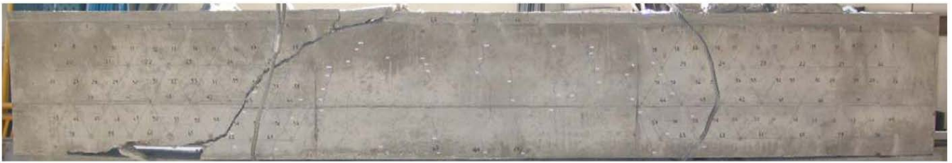
Figure 3. View of specimen after failure.
