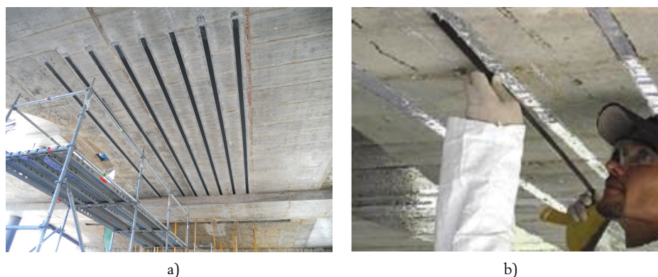
Figure 2. a) Externally bonded reinforcement (courtesy of Mapei), b) Near surface mounted reinforcement [16].
