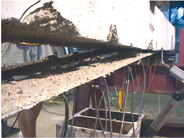
Figure 5. Debonding of the CFRP strengthening system [30].
