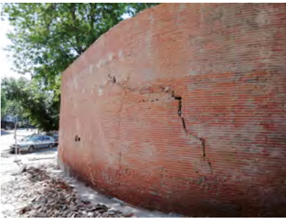
Figure 47. Masonry front wall appearance after plaster removal.
