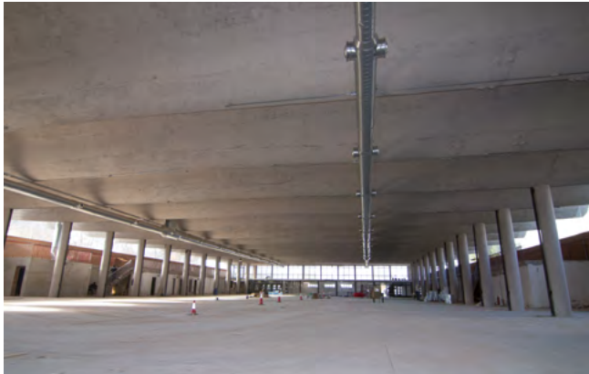
Figure 27. Final state shell roof after rehabilitation.
