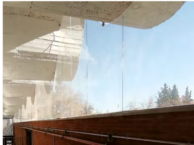
Figure 53. Glass sheets enclosure and fixation to shell roof.
