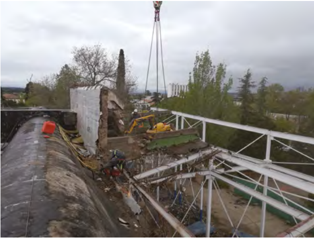
Figure 40. Existing structure demolition.
