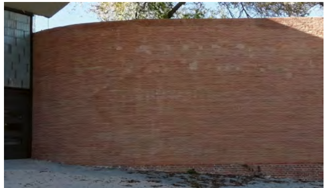
Figure 51. Final appearance of brick walls after rehabilitation.
