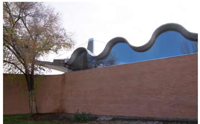
Figure 44. Final appearance of structure and pier top from north façade.
