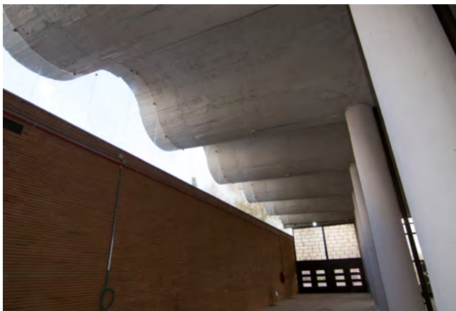
Figure 29. Final state shell roof after rehabilitation.
