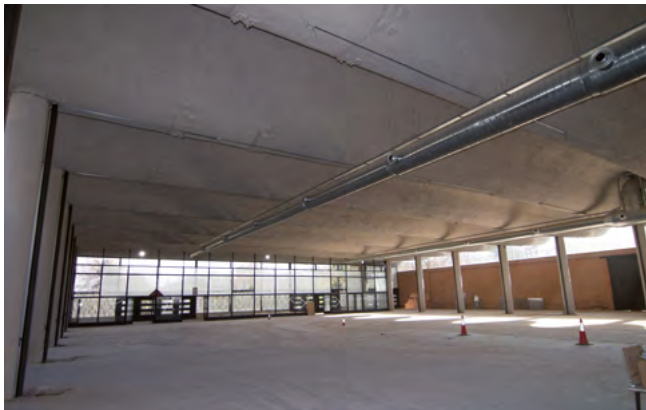
Figure 28. Final state shell roof after rehabilitation.
