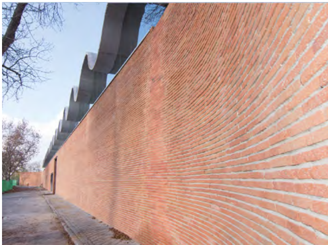
Figure 52. Final appearance of brick walls after rehabilitation.
