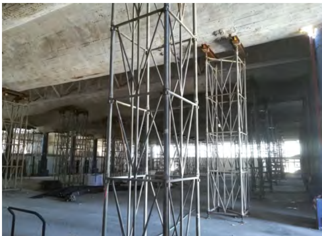
Figure 21. Temporary shoring to ground.
