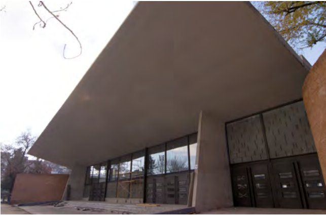
Figure 45. Final appearance of canopy structure.
