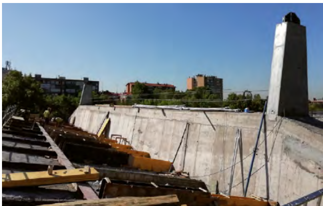
Figure 43. view of concrete box girder and piers after piers concreting.
