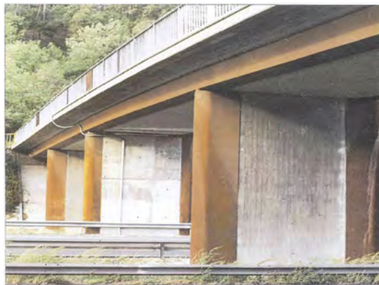
Figure 23. View of the strengthened bridge. Taken from Martínez Calzón [4].
