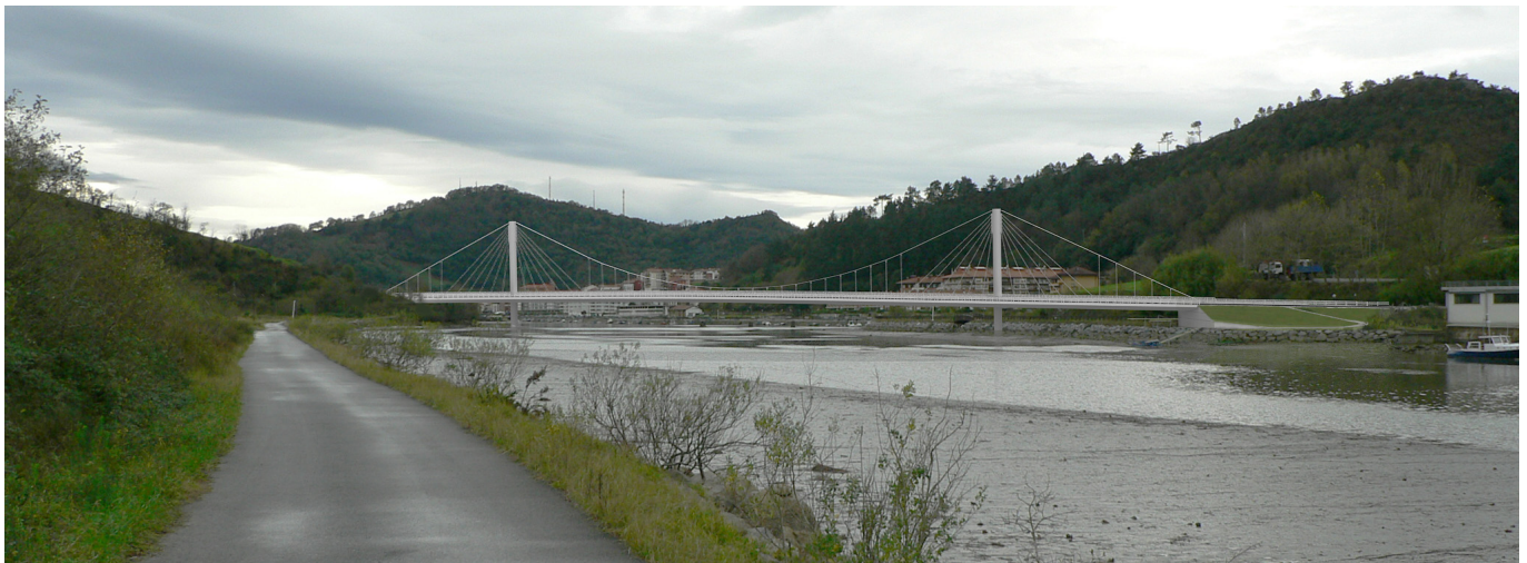
Figure 7. Orio Bridge. (FHECOR).
