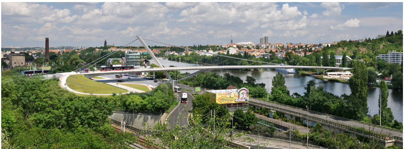
Figure 20. Dvorecky bridge. (FHECOR).
