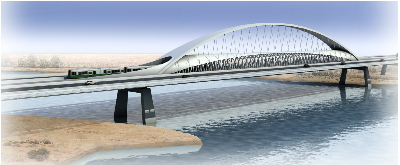
Figure 11. Obhur Bridge. (FHECOR).
