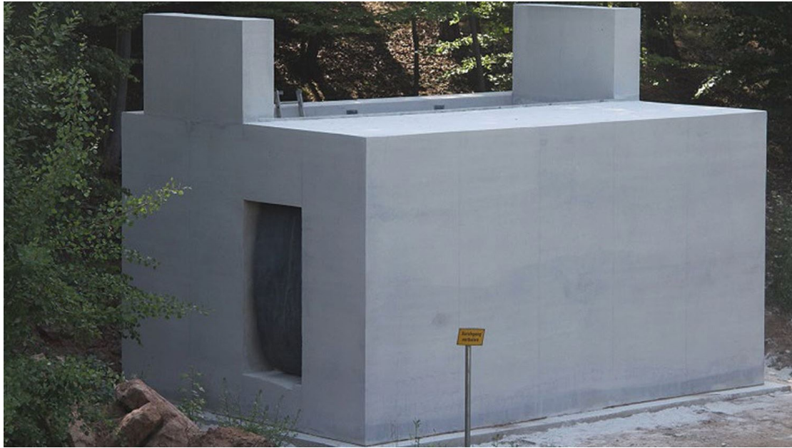
Fig. 10. Experimental building made of Infra-Lightweight Concrete (2014) [10].
