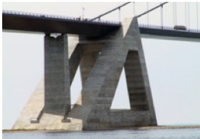
Figure 15. Anchor Block Structure - 1624 m main suspension span.
