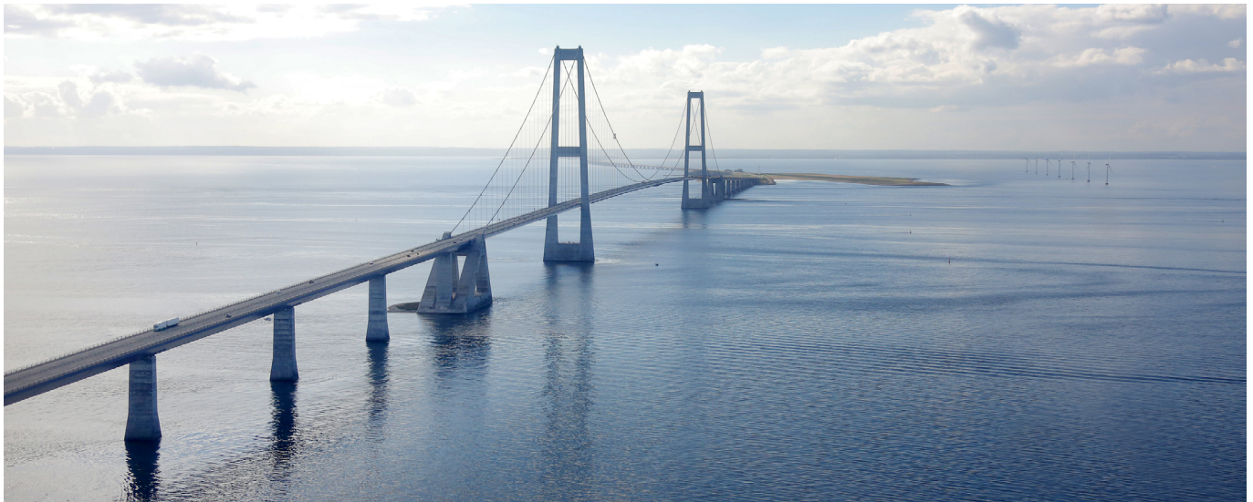
Figure 13. Great belt Suspension Bridge - 1,624 m main span.
