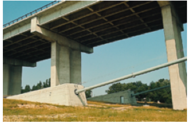
Figure 8. Little Belt Buried Anchorage slab structure.
