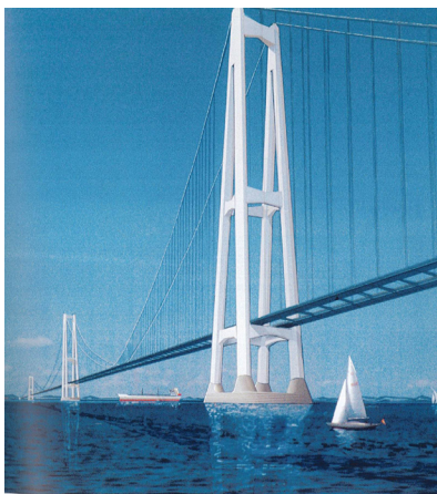
Figure 17. Gibraltar Strait - 3 x 3500 m suspension bridge solution.
