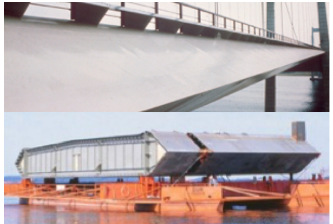
Figure 6. The aerodynamic box girder with wind deflectors.
