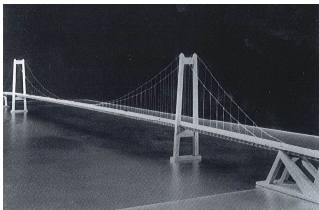
Figure 9. Great Belt rail cum motorway bridge design 1,416 m span.
