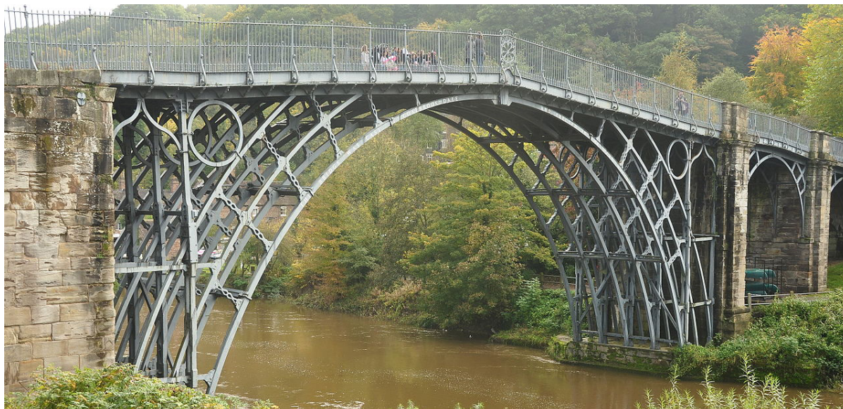
Figure 1. Iron bridge – 60 m.
