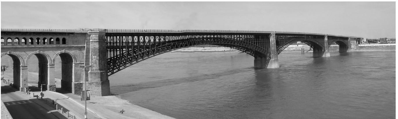
Figure 5. Eads Bridge (1874) – 3 x 158,5 m.
