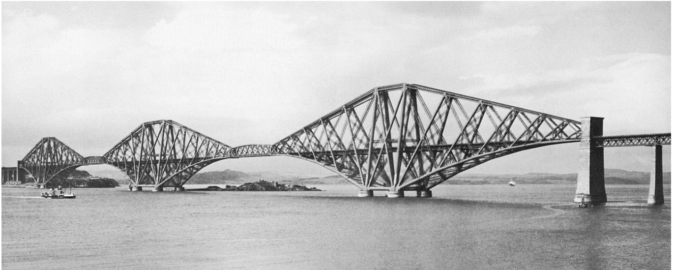
Figure 4. Firth of Forth bridge (1890) – 2 x 521 m.
