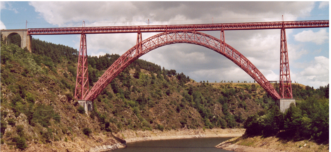
Figure 3. Viaduct of Garabit – 165 m.
