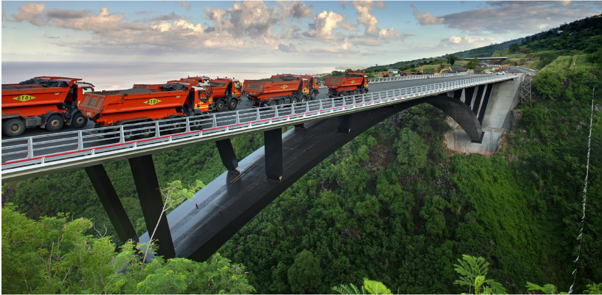
Figure 23. Arch bridge over the Ravine Fontaine.
