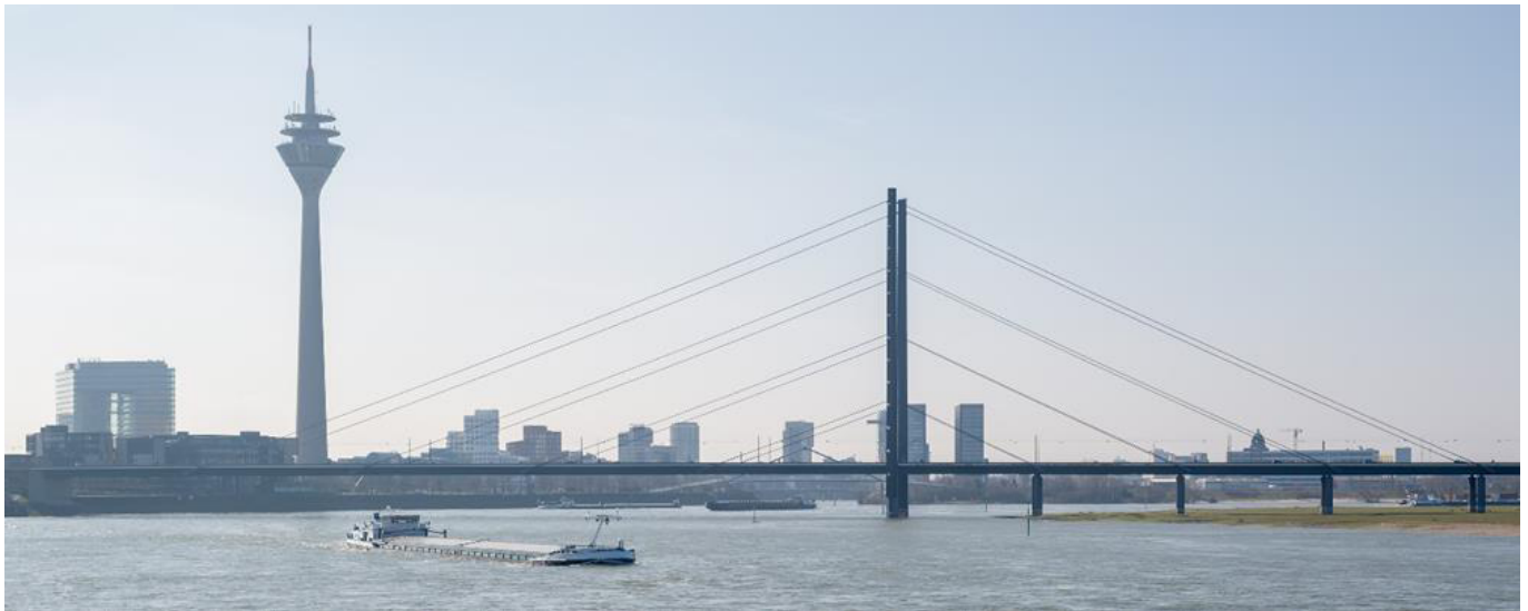
Figure 3. Oberkassel Bridge, Dusseldorf, Germany.
