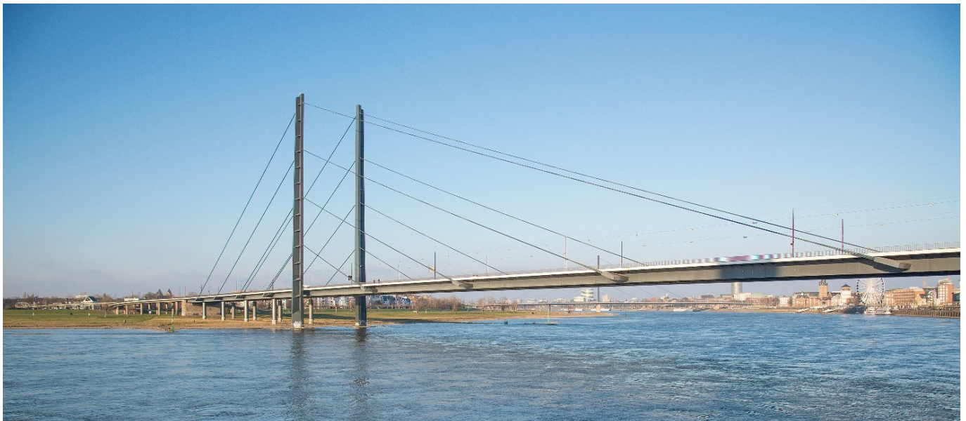
Figure 2. Knie Bridge, Dusseldorf, Germany.
