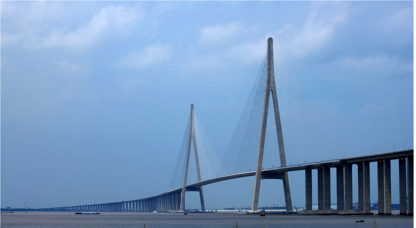
Figure 15. Sutong Bridge, China.
