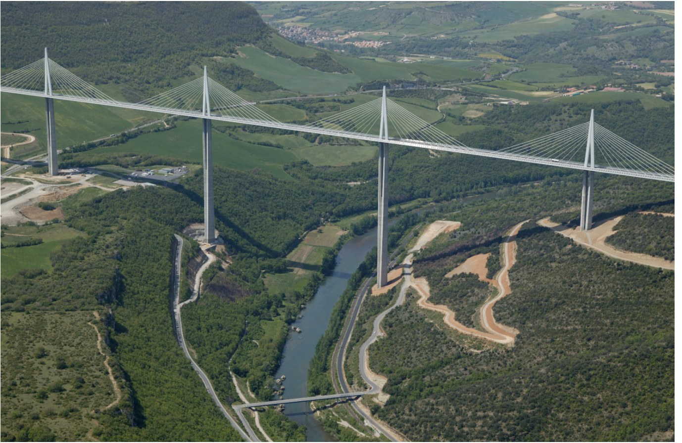
Figure 25. Millau Viaduct, France.
