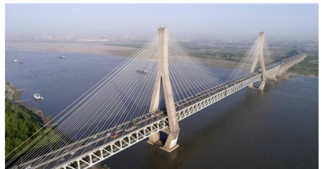
Figure 18. Tiangxingzhou Bridge, Wuhan, China.
