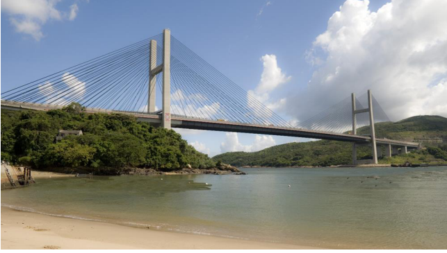
Figure 13. Kap Shui Mun Bridge, Hong Kong.
