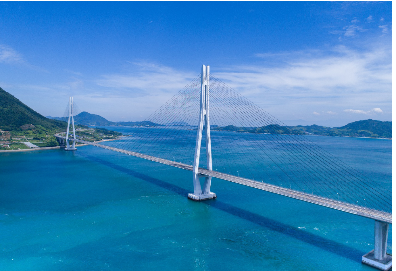
Figure 12. Tatara Bridge, Japan.
