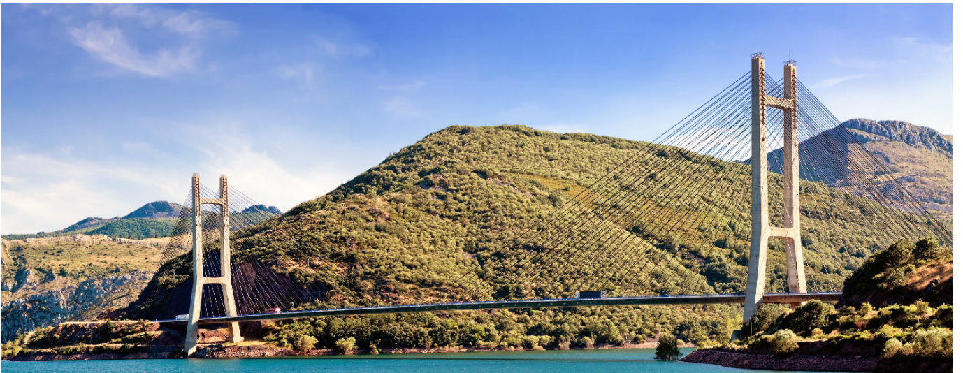
Figure 7. Barrios de Luna Bridge, Spain
