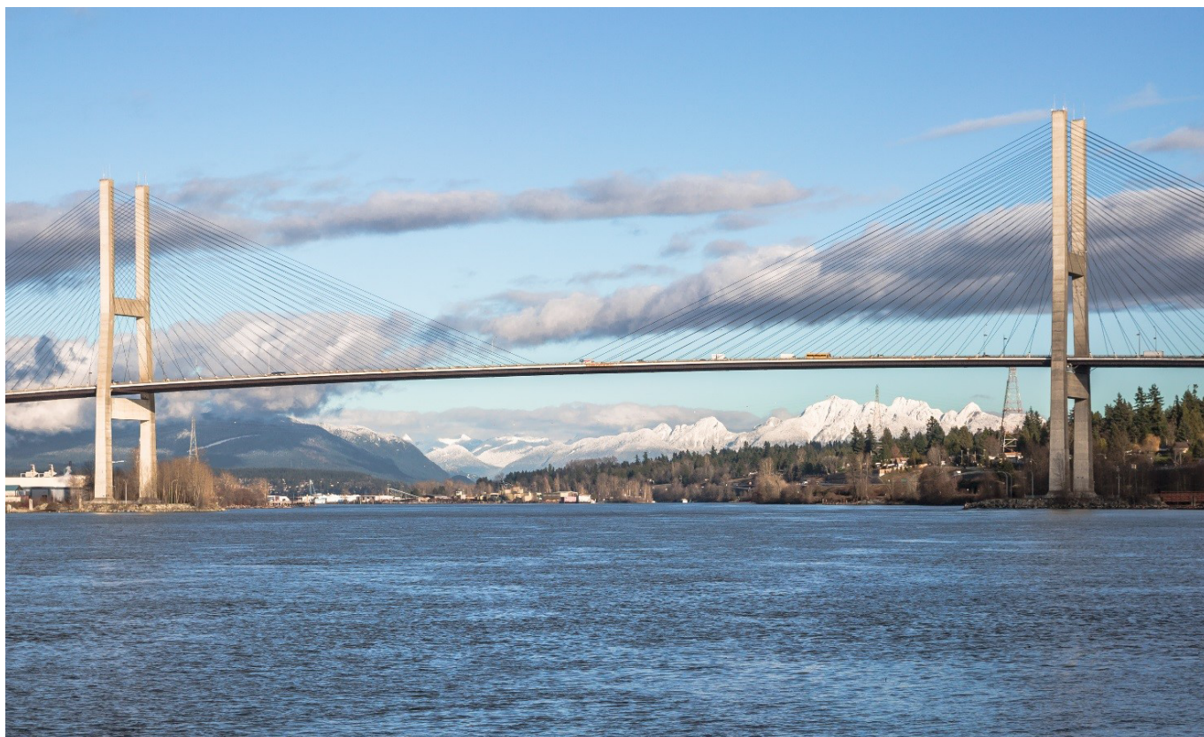
Figure 8. Alex Fraser Bridge, Vancouver, Canada.
