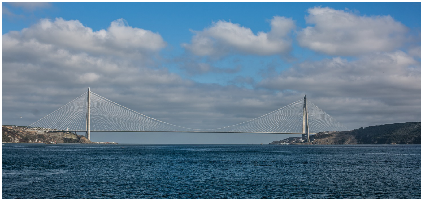
Figure 27. Yavuz Sultan Bridge, Istanbul, Turkey.
