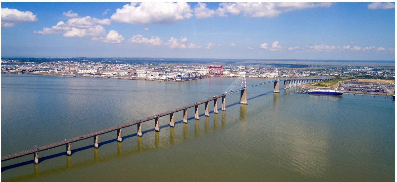
Figure 4. St. Nazaire Bridge, France.
