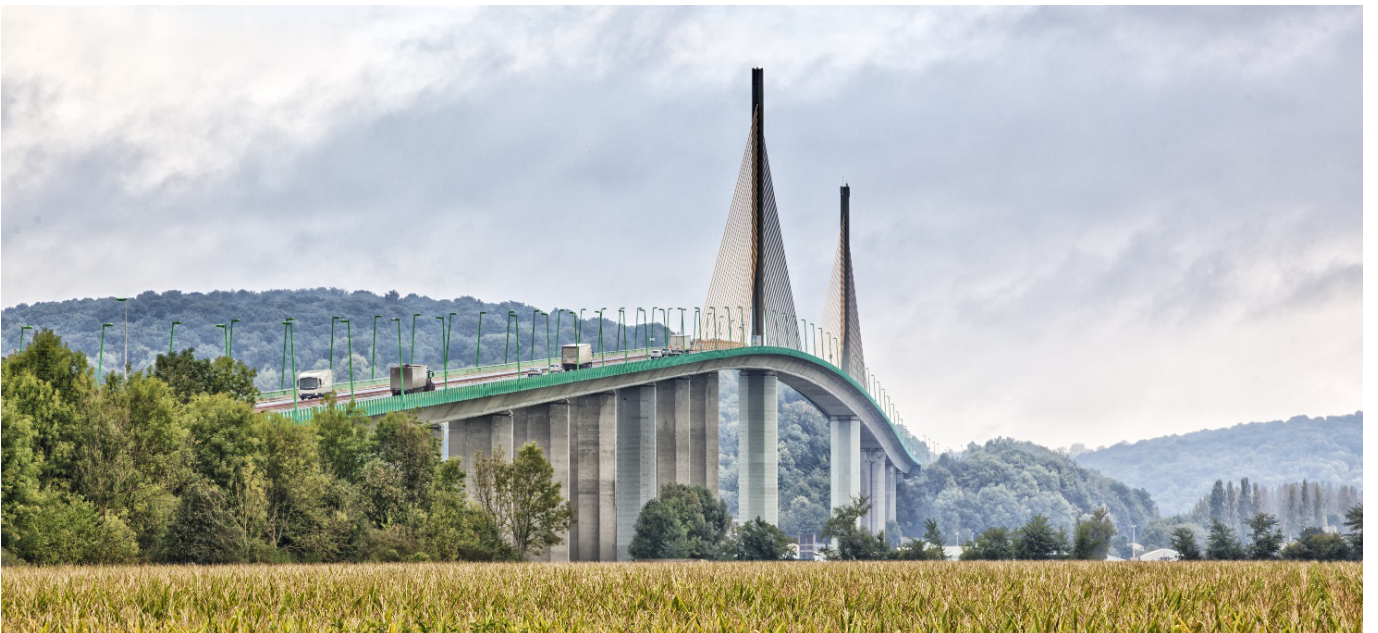
Figure 6. Brottonne Bridge, France.
