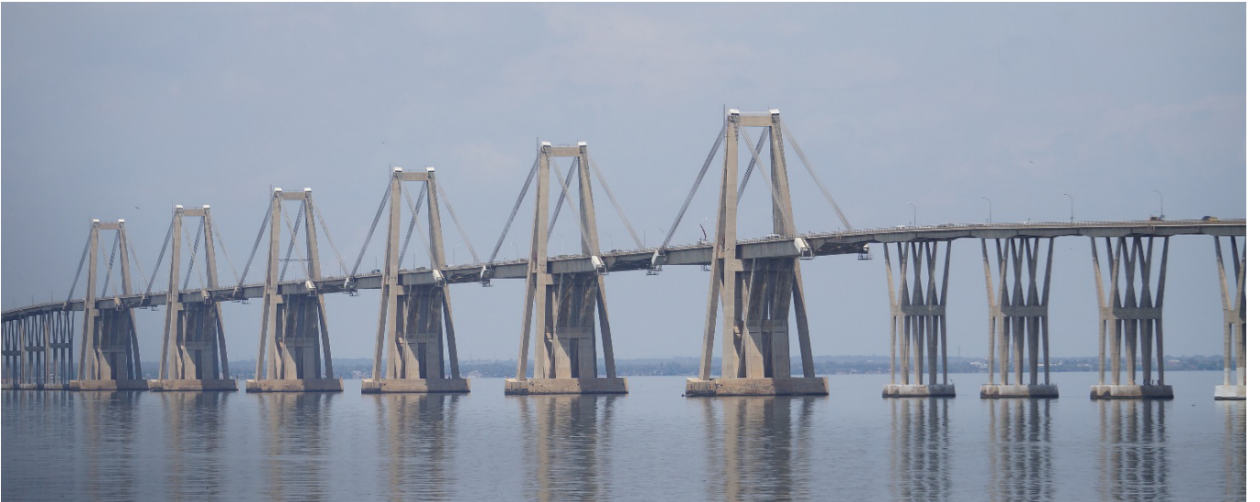
Figure 5. Maracaibo Bridge, Venezuela.
