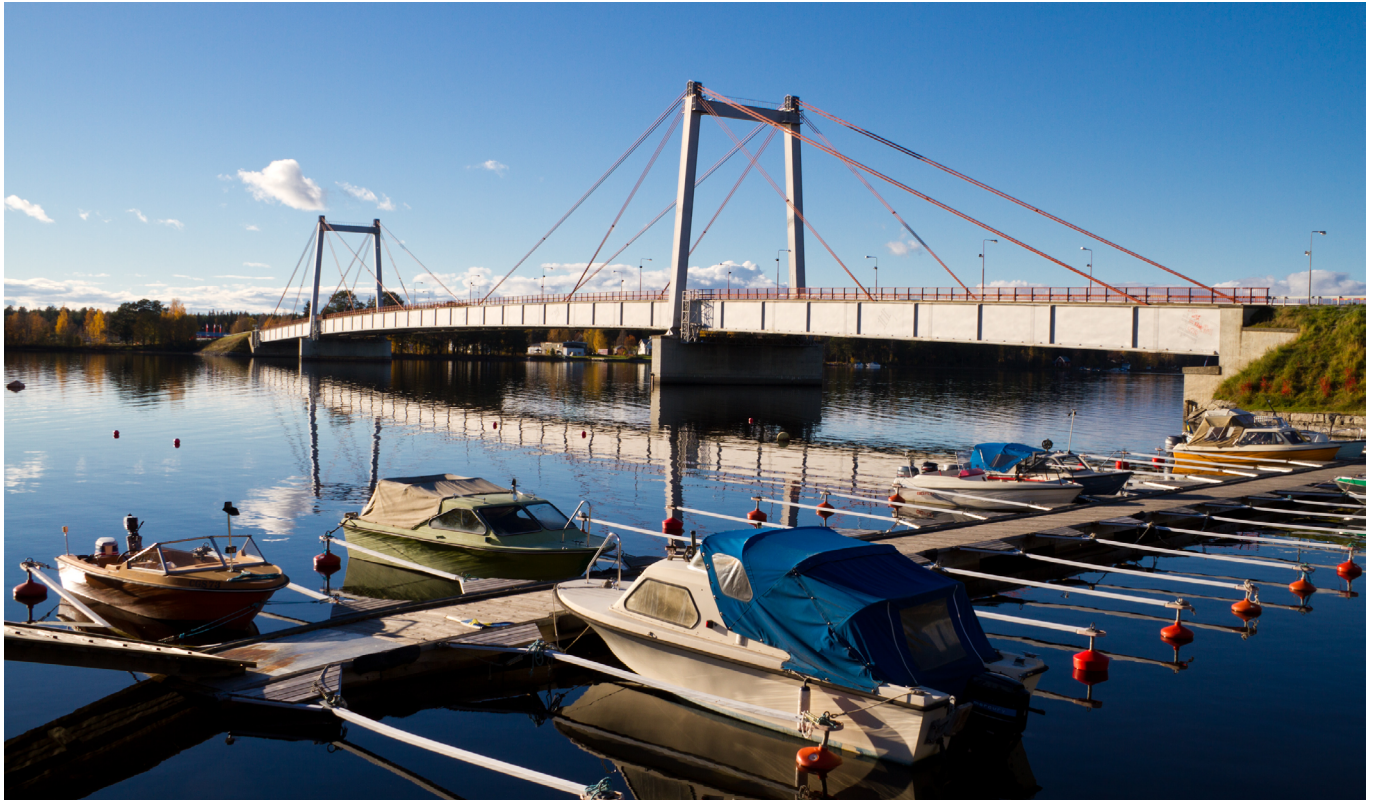
Figure 1. Stromsund Bridge, Sweden.
