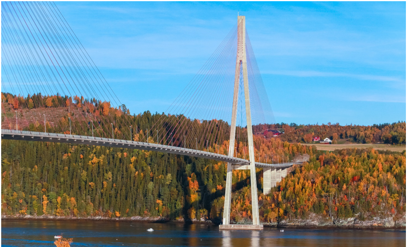
Figure 9. Skarsundet Bridge, Trondheim, Norway.
