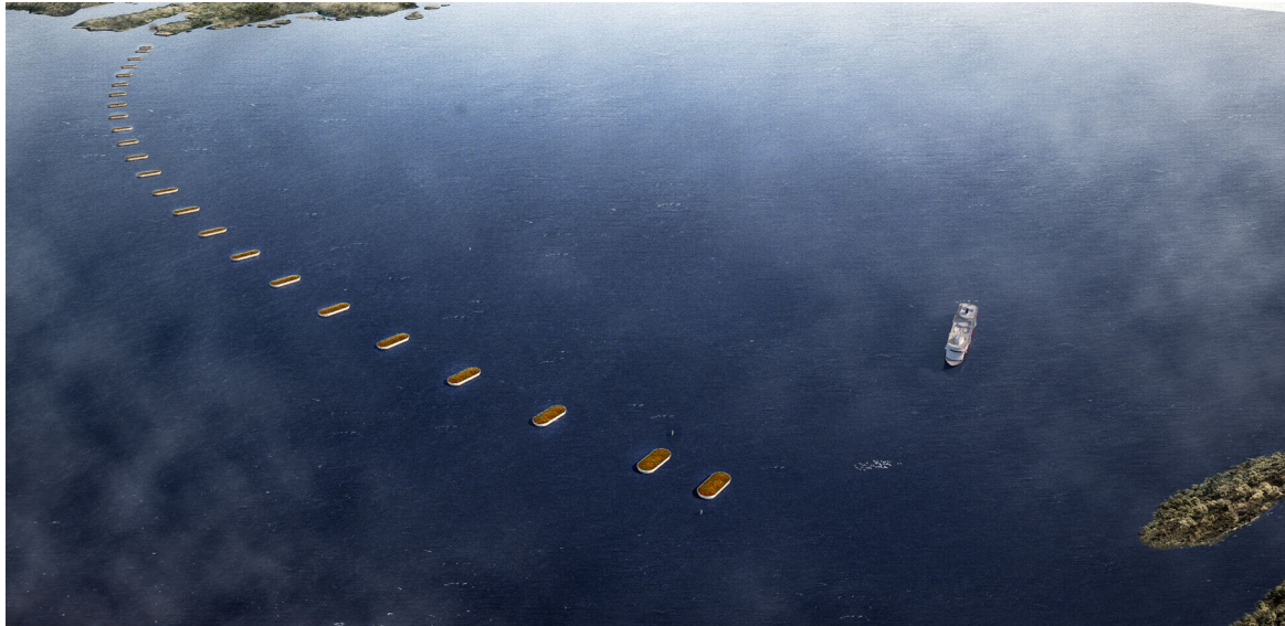
Figure 7: study for an SFTB with pontoons for the Bjørnafjord crossing in Norway, Statens vegvesen
