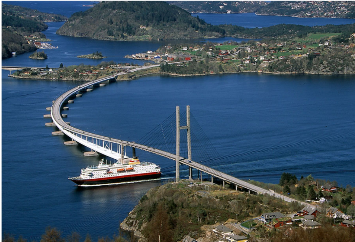
Figure 2: Nordhordland bridge – Aas Jakobsen
